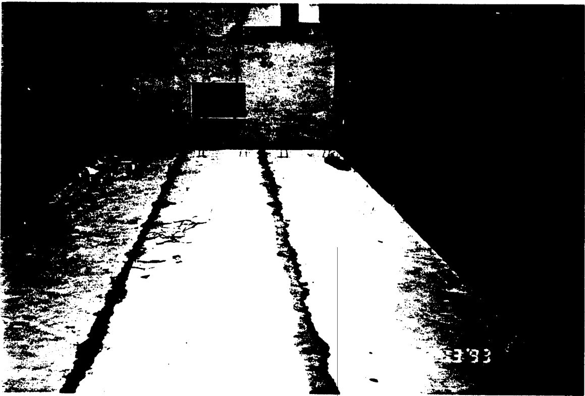
Fig 7.13 The two longitudinal joints filled with mortar
