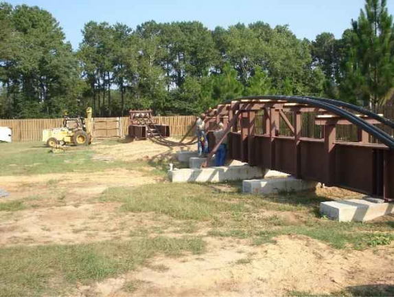
Figure 5-10 HDPE duct on the support frame after welding
