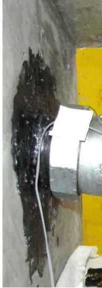
Figure 6-43 Sealant placed on concrete around HDPE pipe
