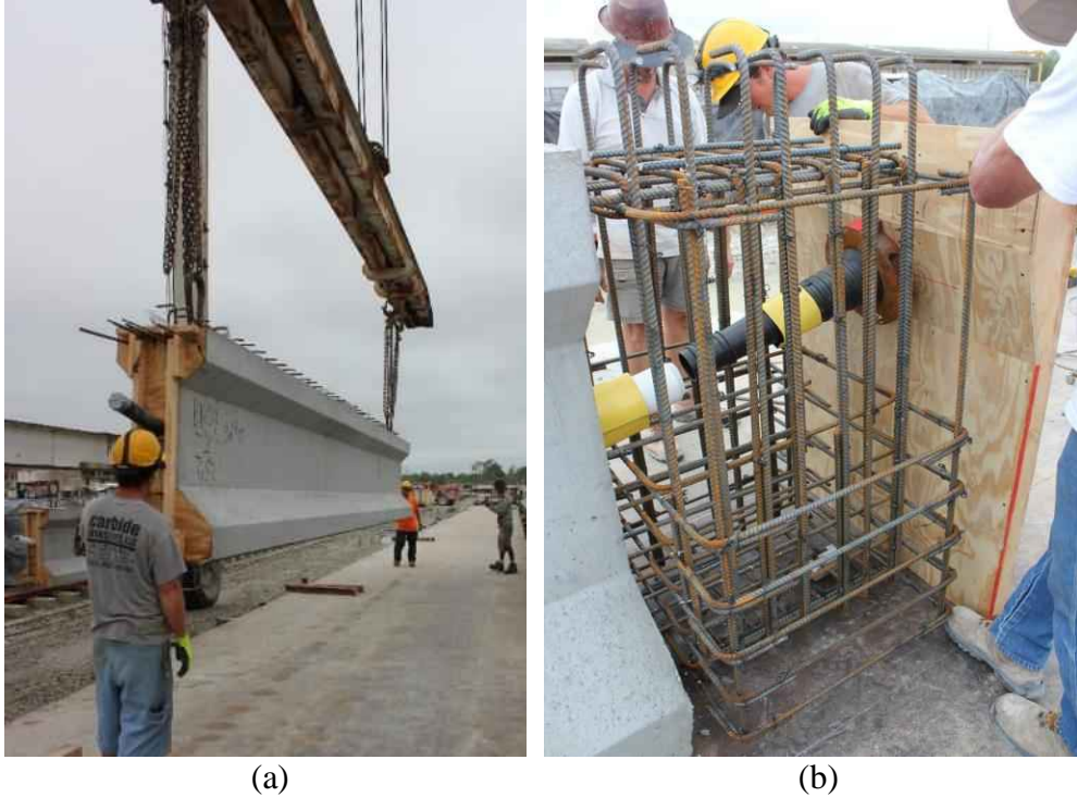
Figure 6-4 Specimen construction: (a) main span, (b) endblocks
