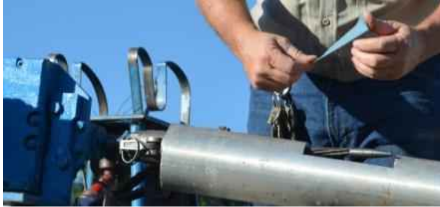
Figure 5-15 Bullet on the head of the strand during pushing
