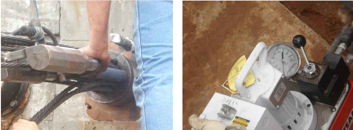
Figure 5-18 Monostrand hydraulic jack and pump used to stress strands
