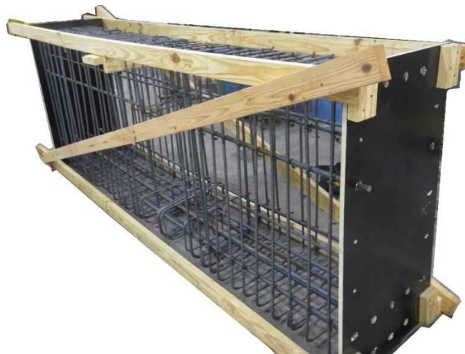
Figure 6-25 Reinforcing bar cage
