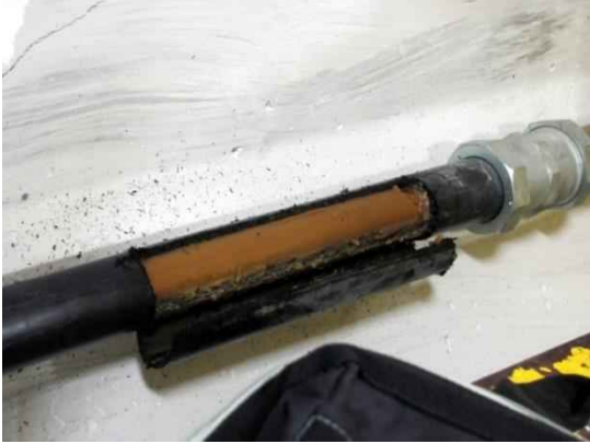
(a) exposing the duct to access the strands
