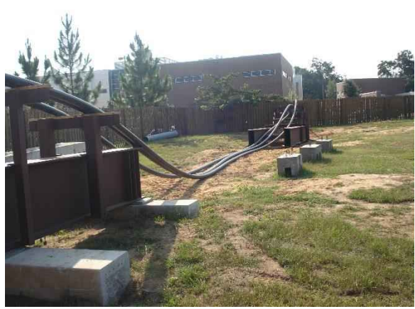
Figure 5-10 HDPE duct on the support frame after welding
