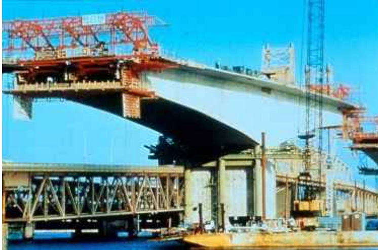
Figure 4-4 Form travelers (Corven J. and Moreton A 2004)
