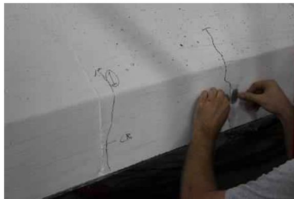
Figure 5-5 Crack opening gage installation
