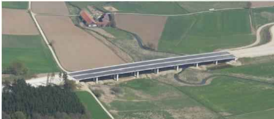
Figure 3-5 Ariel view of Kleine-Laber-Viaduct (Traute and Weiher 2011)
