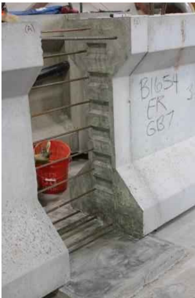
Figure 4-7 Shear keys and protruding reinforcement
