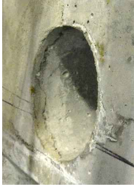
Figure 13-14 Concrete repair for specimen F1 at the end of cyclic loading
