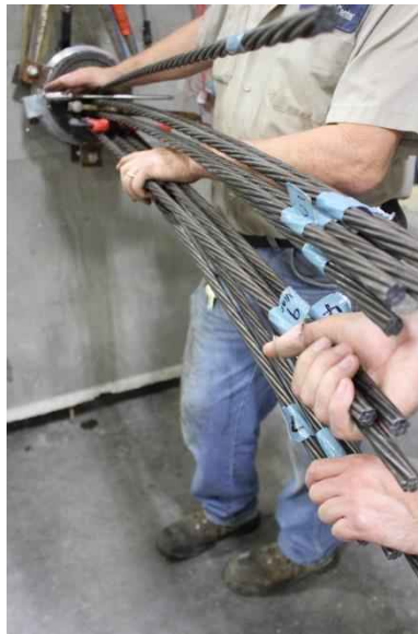
Figure 6-6 Strand pushing
