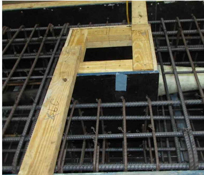
Figure 4-21 General zone reinforcement at hollow section
