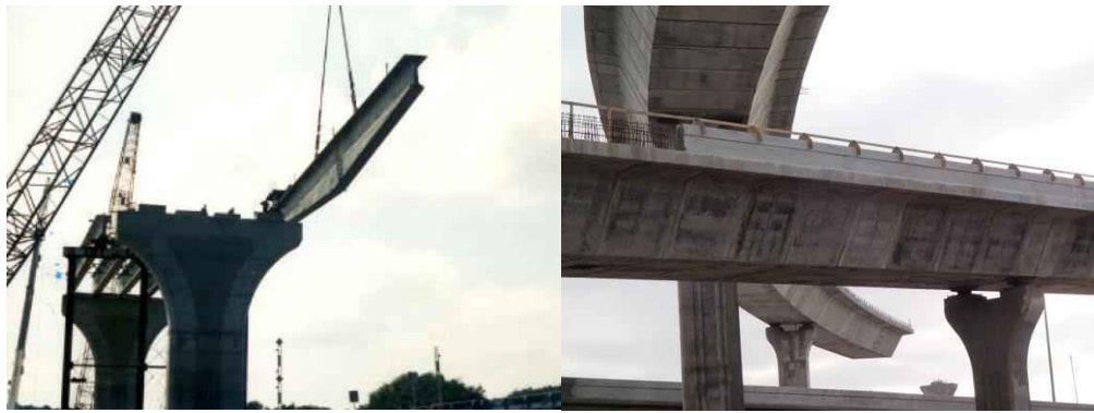
Figure 2-2 Segmental and I-girder bridge construction (FDOT 2002)
