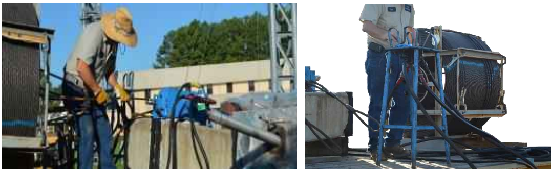
Figure 5-14 Strand installation using Model 00143604/2 strand pusher from PAUL Maschinenfabrik GmbH & Co
