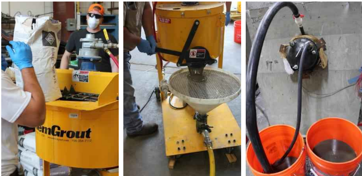
Figure 6-10 Grouting operation: (a) feeding hopper, (b) uniform consistency, (c) at outlet
