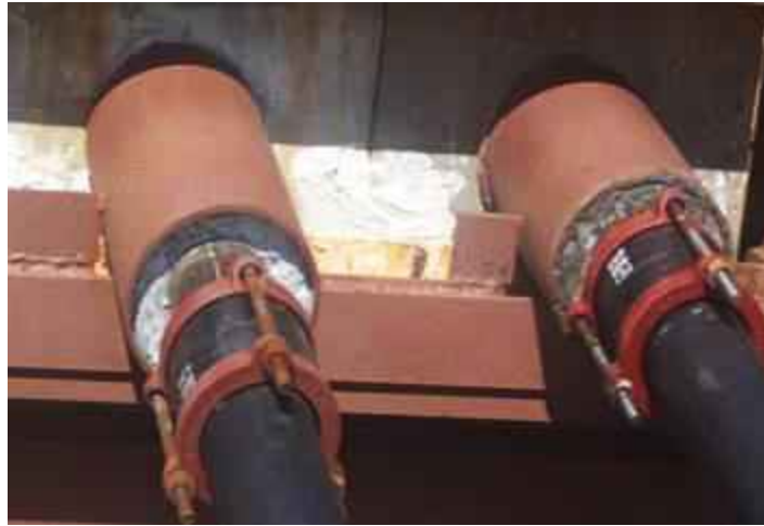
Figure 5-13 West end connected to the anchor block
