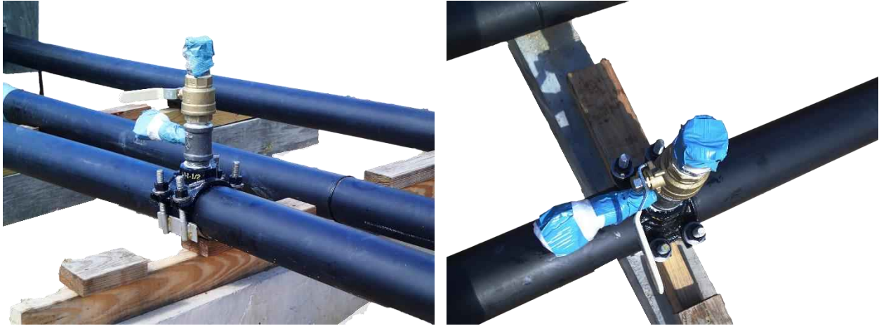
Figure 5-6 Injection into saddle
