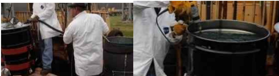
Figure 5-25 Filler heating logistics: (a) transfer of filler between barrels and (b) filler agitation.
