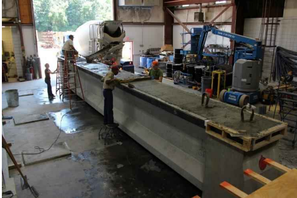
Figure 6-5 Deck casting on internal specimens
