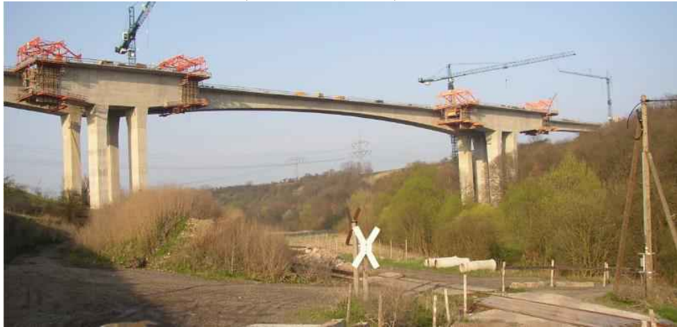
Figure 3-3 Weidatal bridge under construction (Zilch et al. 2007)
