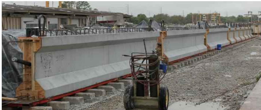
Figure 6-1 Segments in prestressing bed
