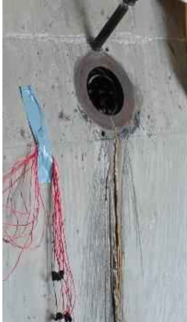
Figure 8-2 End of beam where wedges were torched
