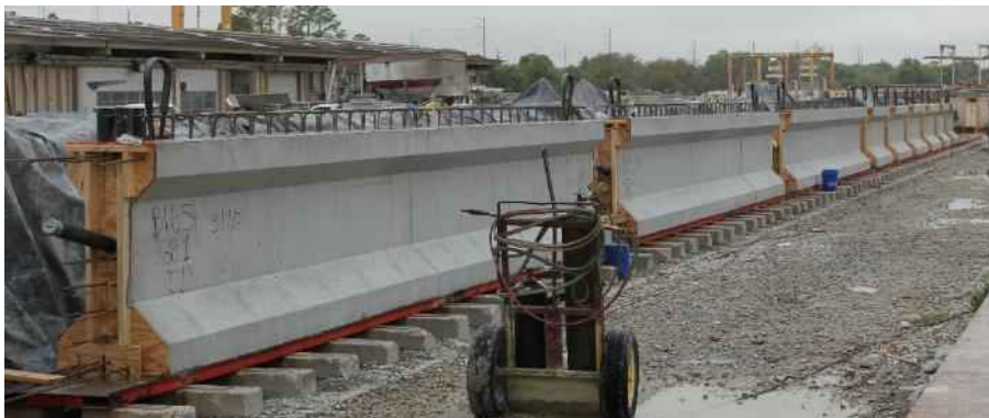
Figure 6-6 Segments in prestressing bed
