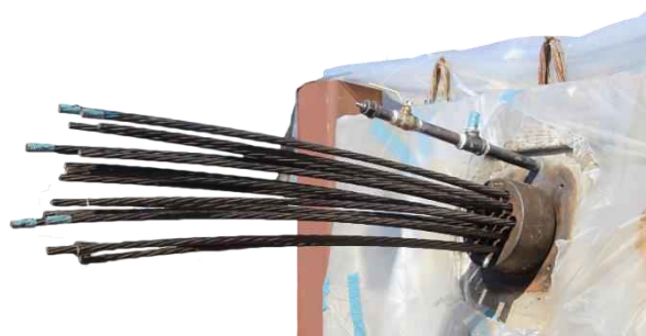
Figure 5-17 Wedge plate installed on anchor
