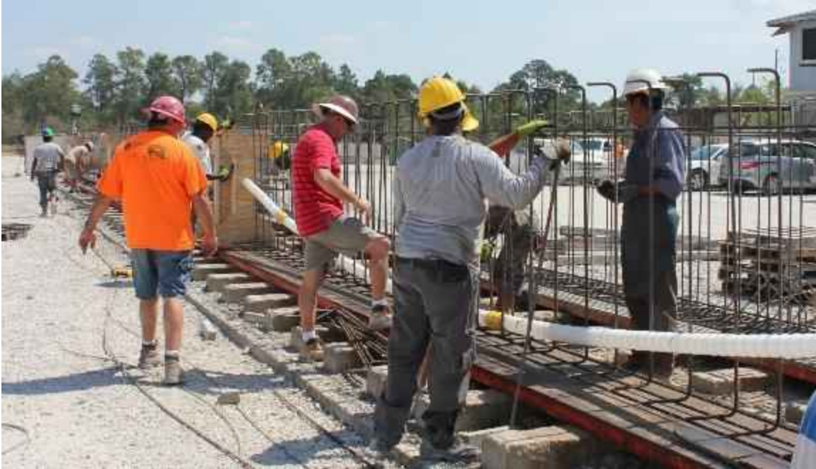
Figure 6-3 Duct installation
