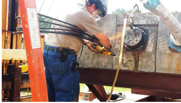
Figure 5-20 Strand tails cutting in operation
