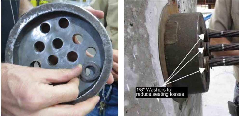
Figure 6-35 Washers to reduce seating losses
