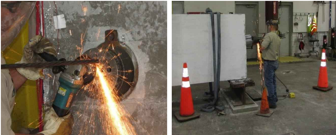
Figure 6-38 Strand cutting after post-tensioning
