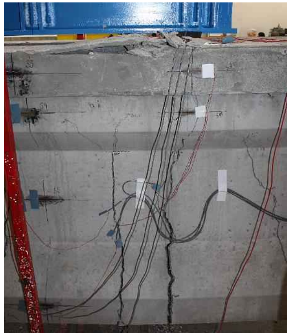
Figure 10-13 IWC: rupture of deck at load point
