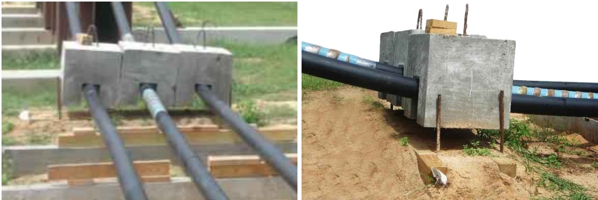
Figure 5-19 Deviators suspended by tendon after stressing
