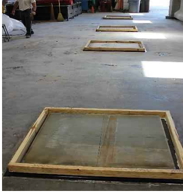
Figure 6-19 Grout pads for deviator blocks
