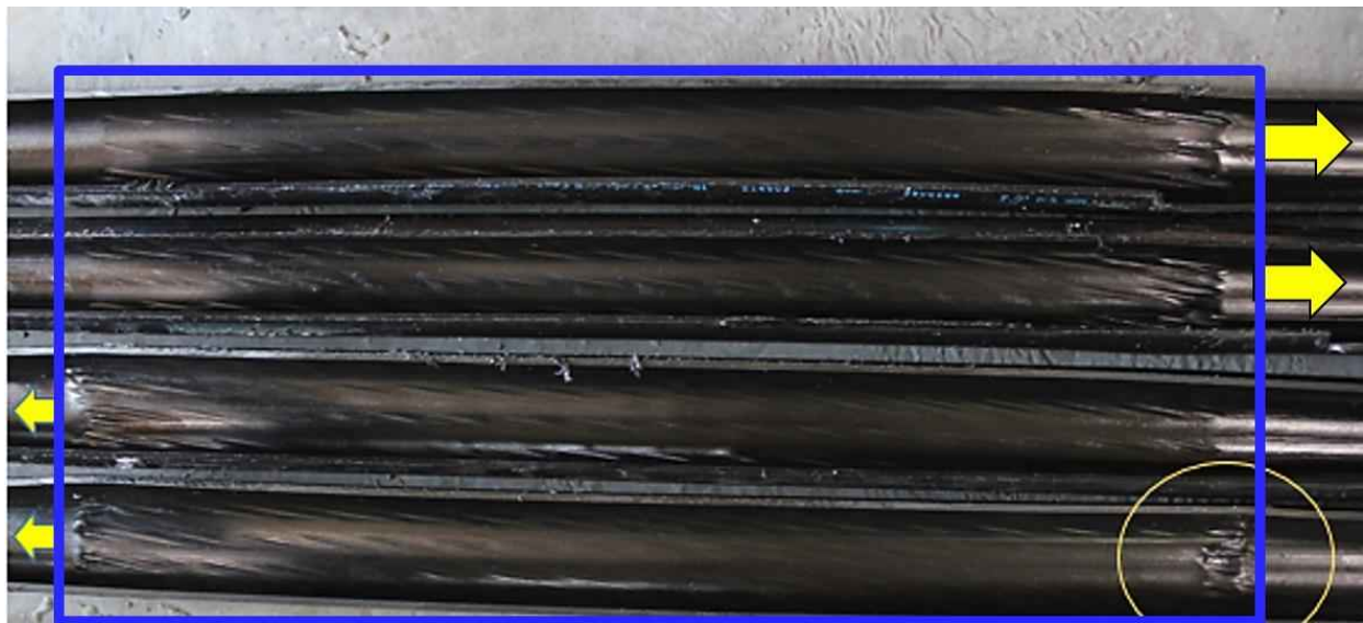
Figure 11-19 EWS: interior surface of duct in contact with strand at diablo
