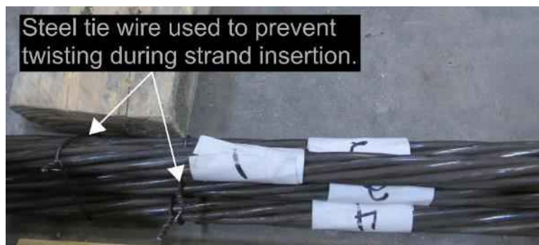
Figure 6-31 Strand labeling and steel ties
