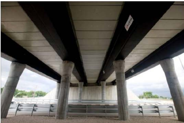
Figure 35. Carbon/glass FRP bridge girder erected in 2007 in Madrid, Spain. Photos from 2012 CICE conference paper by Paulotto et al. [64].
