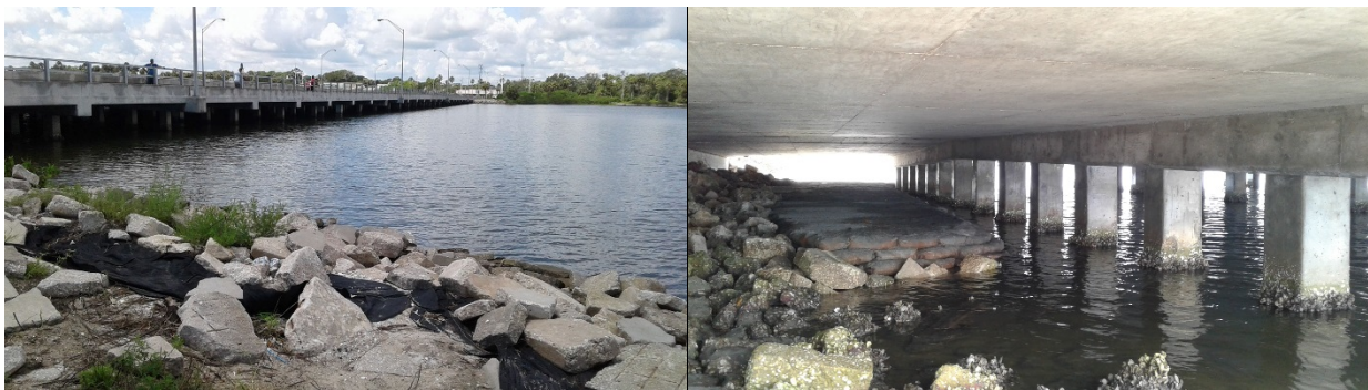
Figure 1. Low-rise relief bridge on Dunlawton Causeway in Port Orange, FL.
