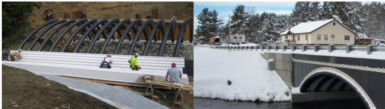
Figure 28. CABS construction and finished bridge.
