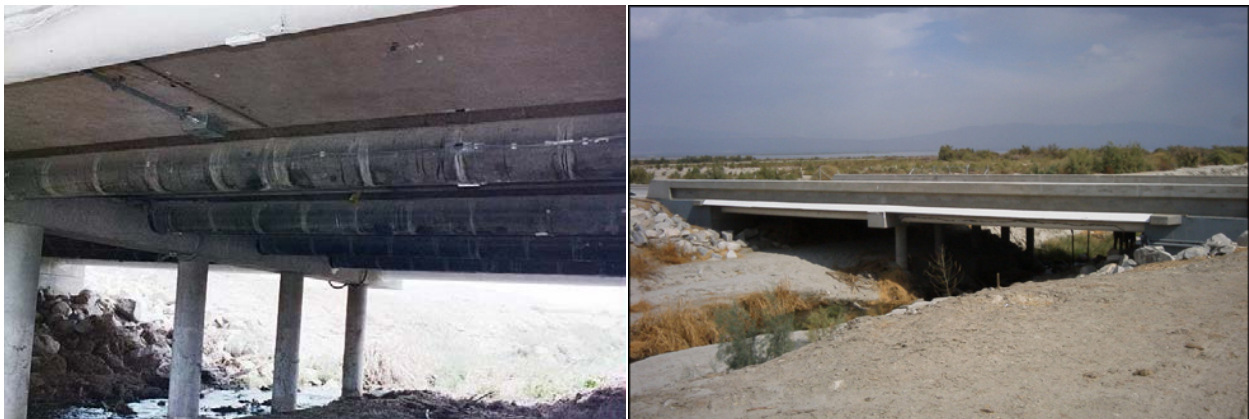
Figure 31. King's Stormwater Channel bridge. California State Highway 86 near the Salton Sea.
