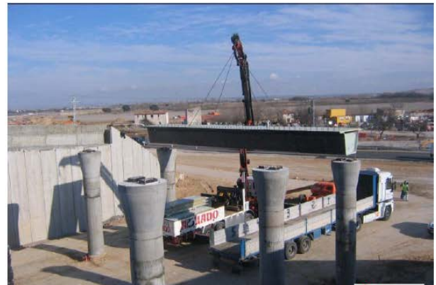
Figure 35. Carbon/glass FRP bridge girder erected in 2007 in Madrid, Spain. Photos from 2012 CICE conference paper by Paulotto et al. [64].
