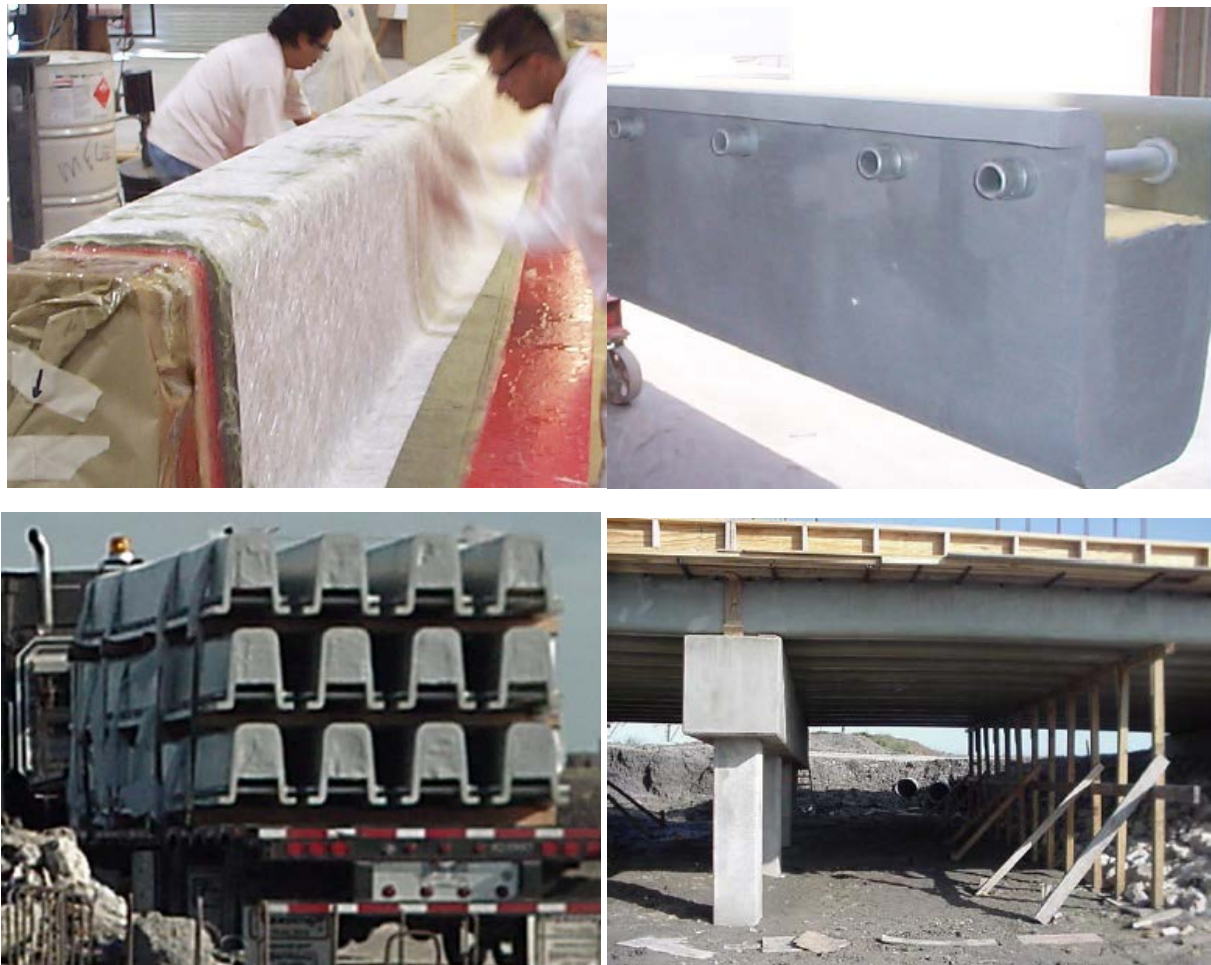
Figure 26. FRP U-Girders for FM 3284 bridge in San Patricio County, TX [52].
