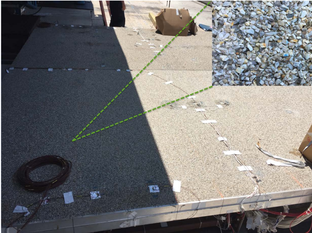
Figure 1. Aluminum bridge deck with a close up view of the aggregate.
