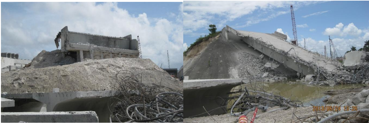
Figure 3-11: Remaining structure after bridge demolition.
