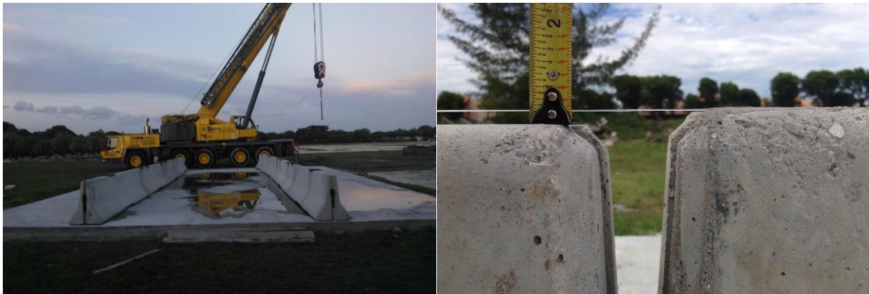
Figure 3-13: Concrete barriers to serve as pedestal for bridge segments.
