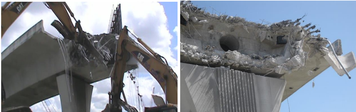
Figure 3-8: Concrete crusher demolition procedures.
