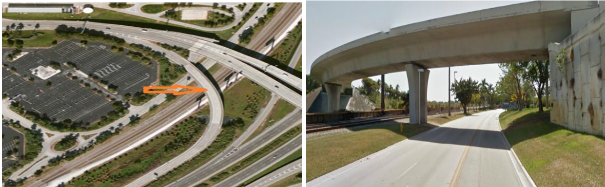
Figure 3-1: A bird's eye view of the exit ramp (left) and side view of bridge (right).
