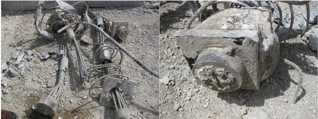
Figure 3-10: Post-tensioning anchor and strands after demolishing of the bridge.
