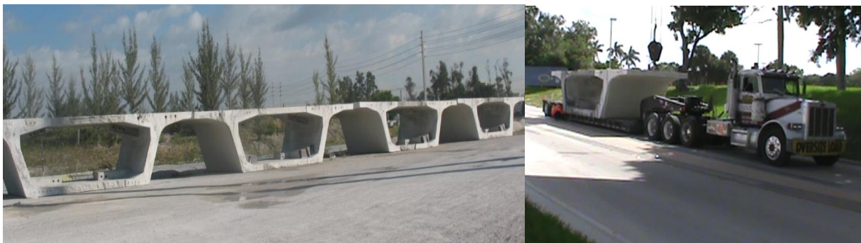
Figure 3-12: Storage of segments at Titan America yard (left) and transport to FIU (right).
