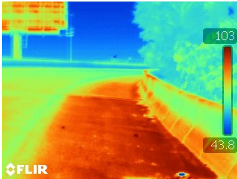
Figure 4-15: Typical infrared image on bridge deck.
