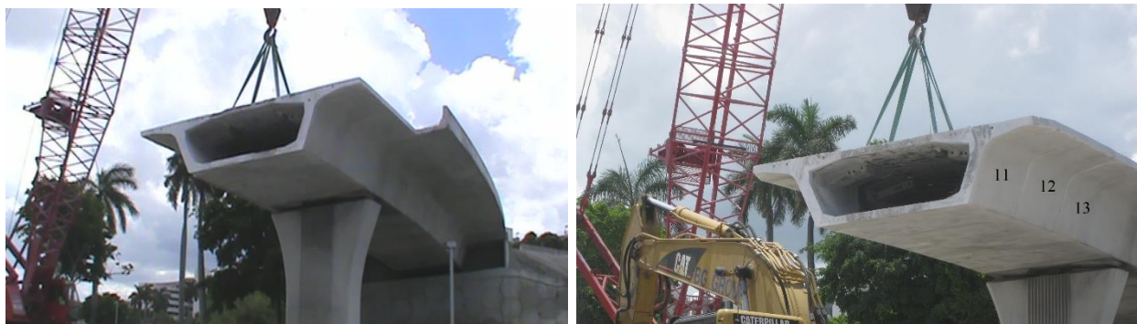
Figure 3-6: Piece-by-piece removal of segments.
