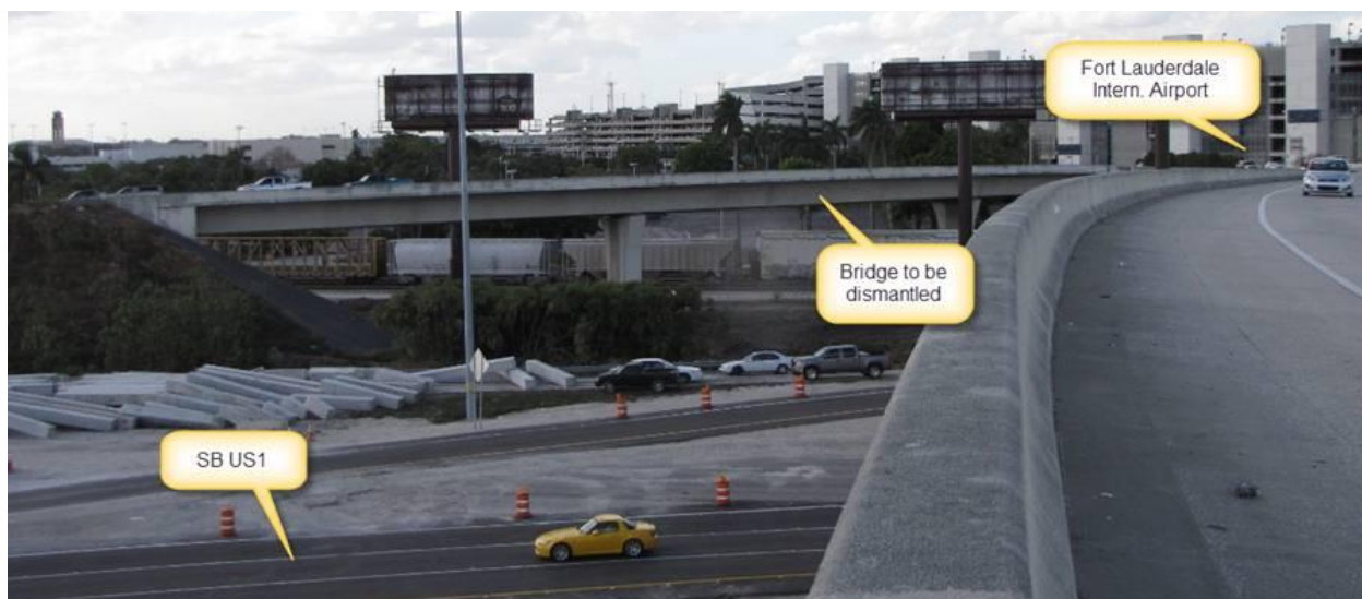
Figure 2-1: Bridge at Fort Lauderdale exit ramp to SB US-1.
