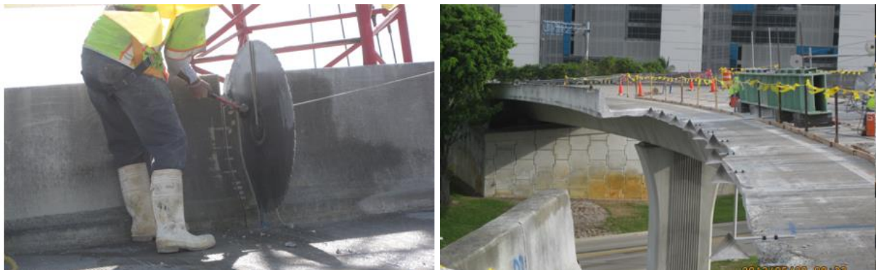
Figure 3-4: Cutting off box wings on both side of the bridge.
