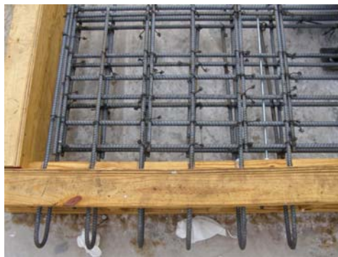
Figure 10 - The hoop bars (4D) in form.
