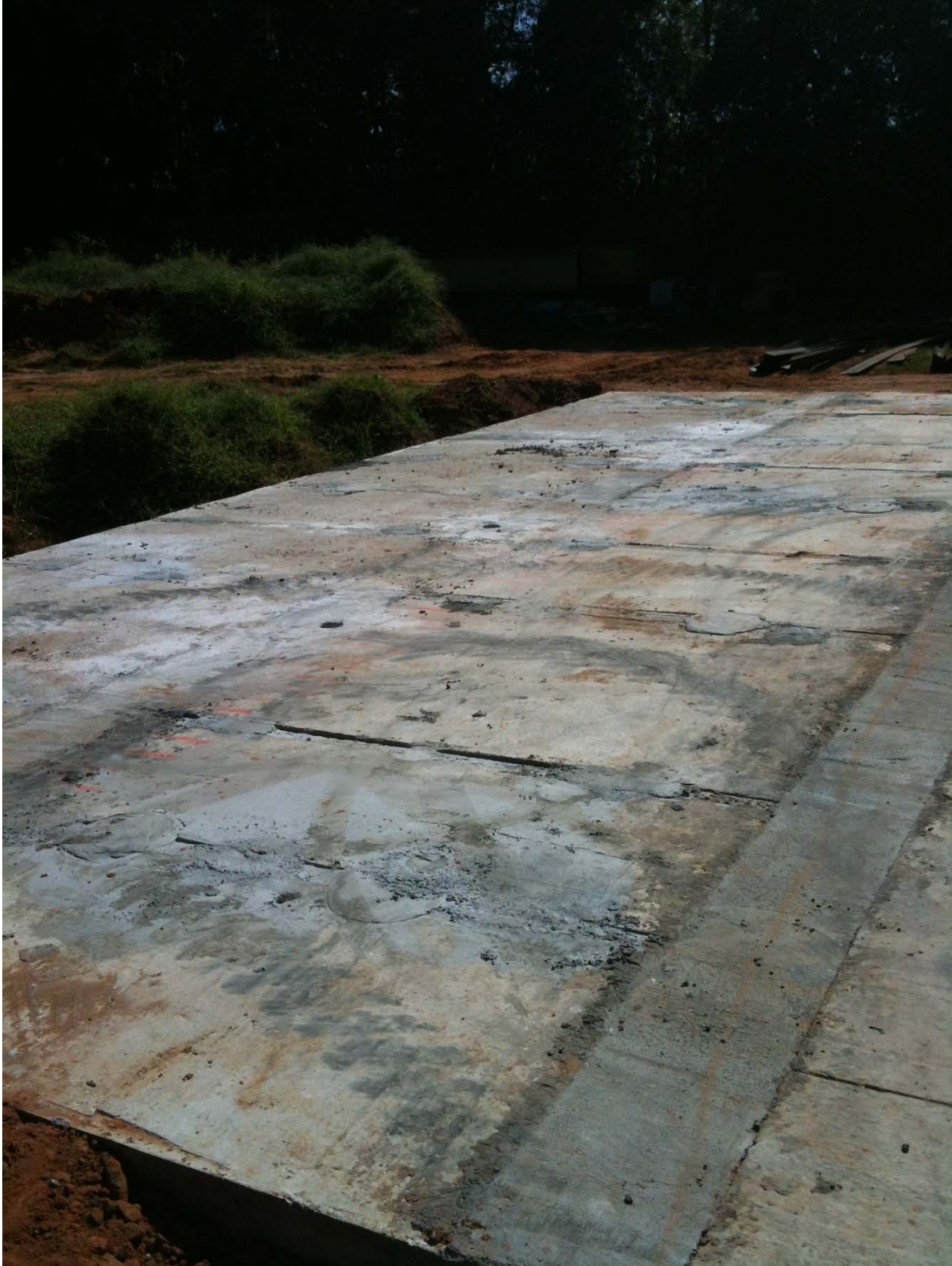
Figure 23 - Completed Full Depth Precast Panel Mock-Up
