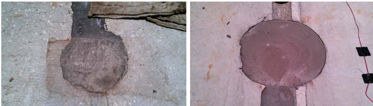
Figure 20 - Grouted shear pockets; Day 1 on left and Day 2 on right
