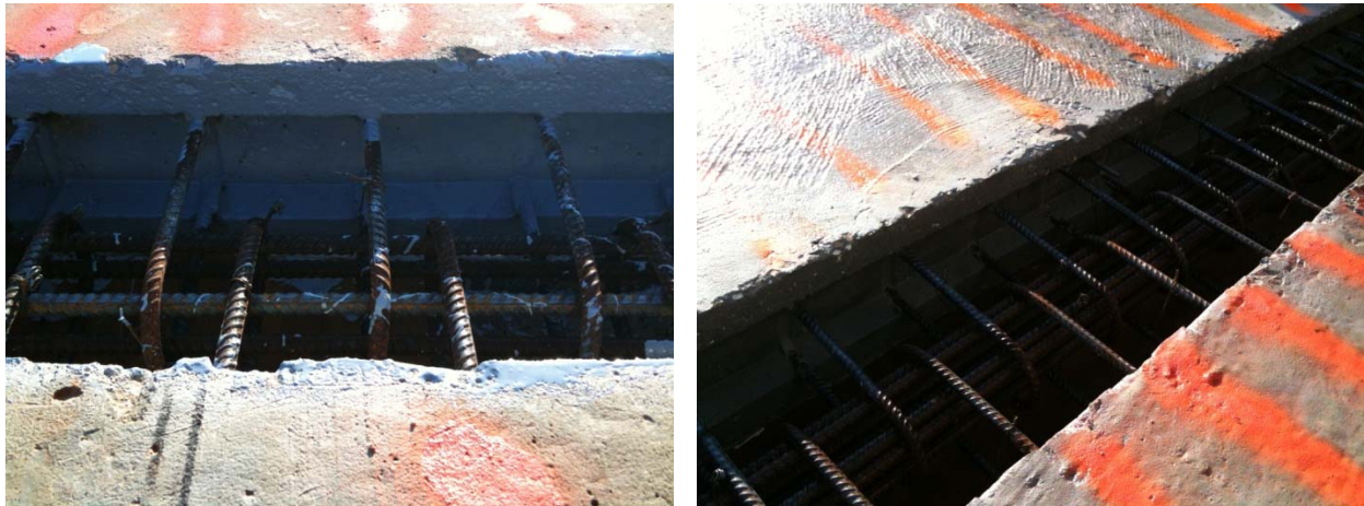
Figure 21 - Epoxy (left) and SSD (right) Keyways
