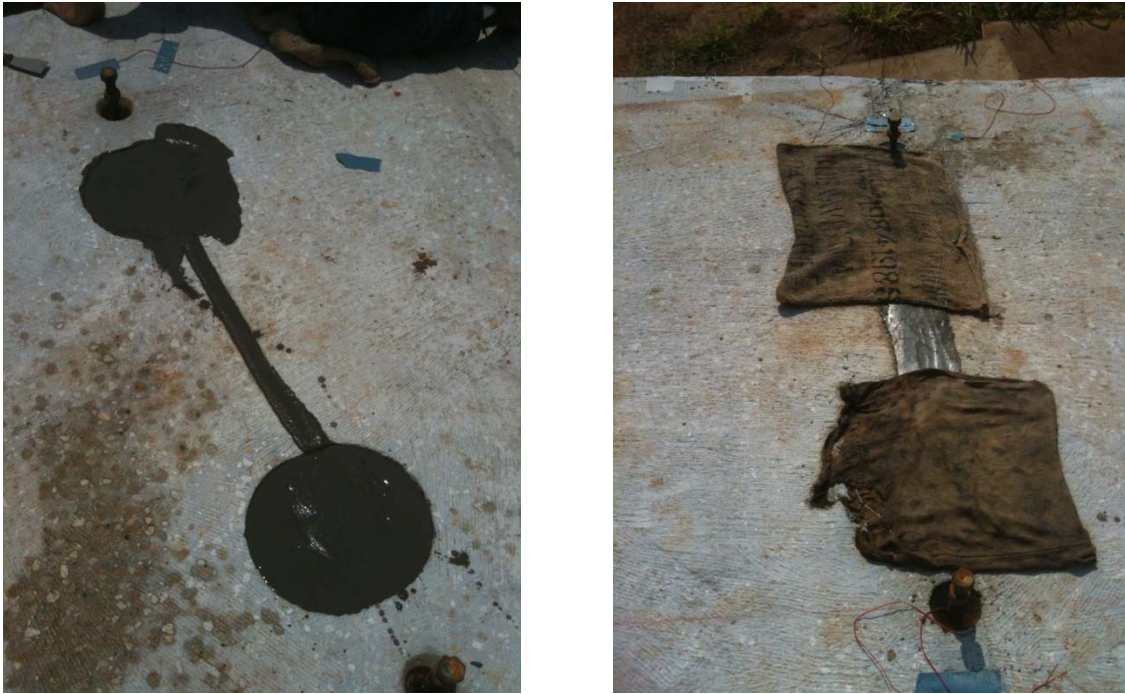
Figure 19 - Day 1 Grout Installation
