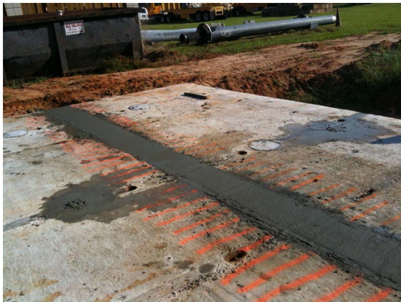
Figure 22 - Transverse Closure Joint
