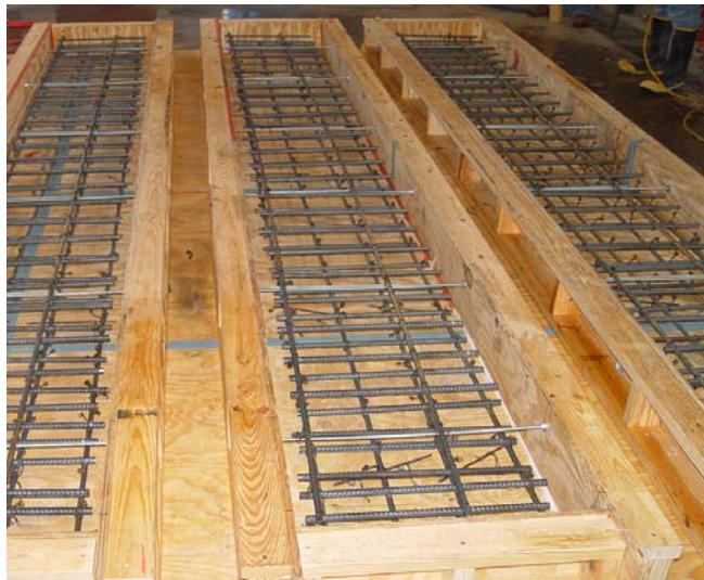
Figure 30 – Forming Panel Specimens with No Joint
