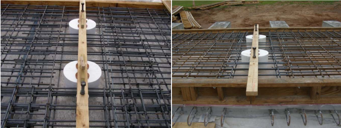
Figure 9 - Splice at midspan of panels. East panel with mild reinforcement (left), West panel with WWR (right).
