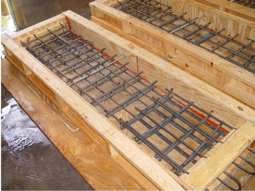
Figure 31 - Forming Panel Specimens for Lapping Hoop Joint
