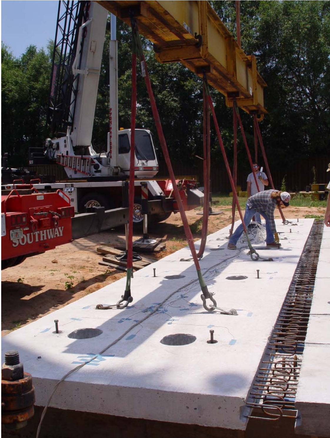
Figure 17 - Hand tightening the bolts during Leveling on Day 2.
