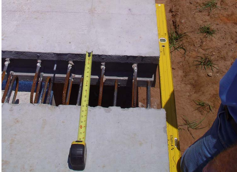
Figure 16 - Lining up the panels while maintaining a 12 inch closure pour.
