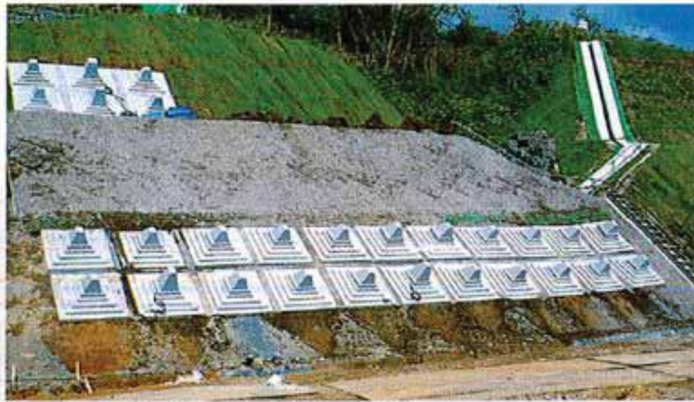
Tendons of the New Material ground anchor "Excellent corrosion resistances and light weight"
