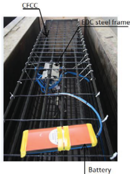
Figure 5.4: EDC installation
