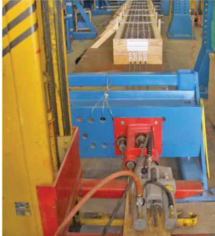
(a) Applying pretension to longitudinal strands
