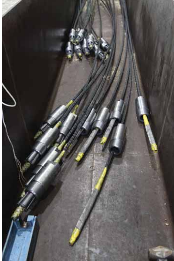
Figure H.17: CFCC coupler installation: several partially-completed couplers in precasting bed
