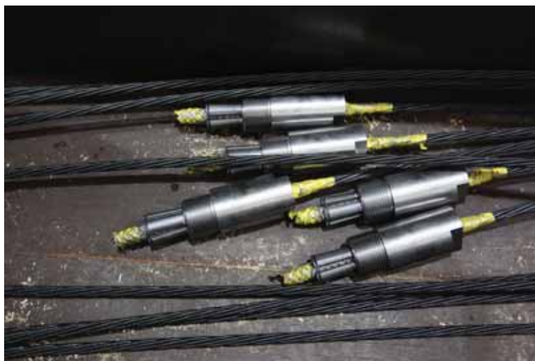
Figure H.19: Partial installation of several couplers
