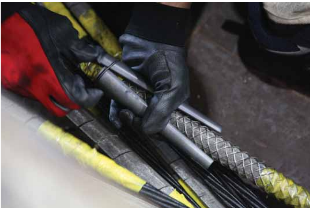
Figure H.10: CFCC coupler installation: placing wedges on mesh-wrapped CFCC strand
