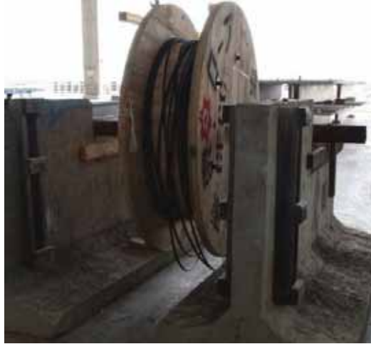
Figure 4.6: Assembly to lay strands
