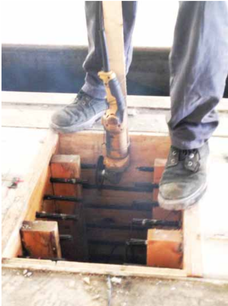
Figure H.30: Cutting CFCC strands with a side grinder
