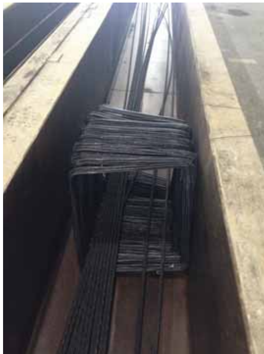
Figure H.4: View of precasting bed, showing bundle of CFCC spirals
