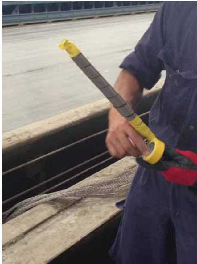
Figure H.8: CFCC coupler installation: wrapping the CFCC strand with mesh
