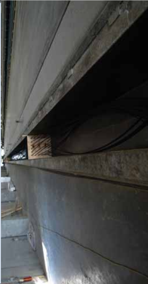
Strands in position. Note the adjacent, previously-cast pile in the self-stressing forms.
