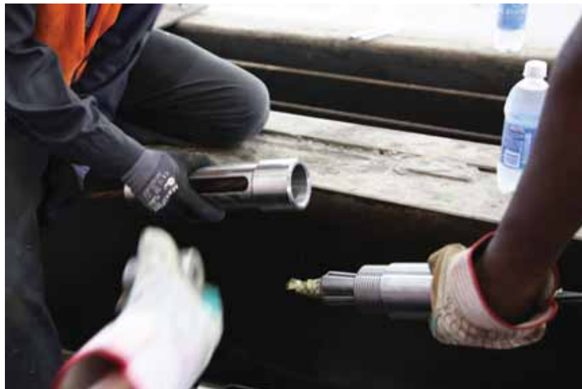
Figure H.14: CFCC coupler installation: ready to screw two parts together
