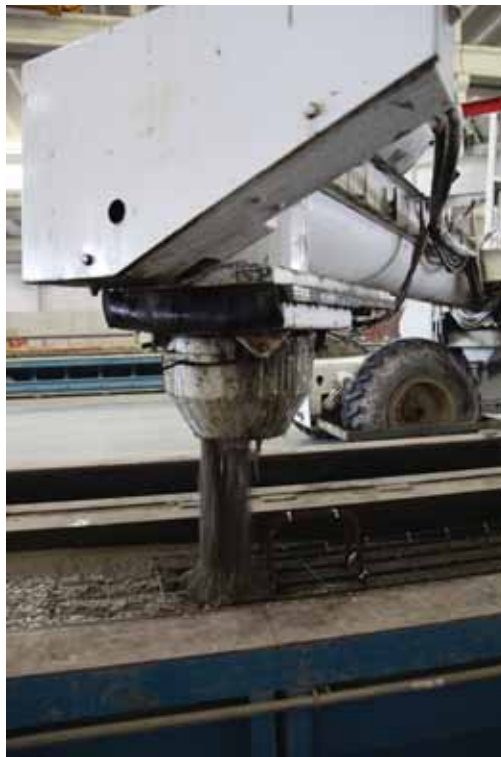
Figure H.27: Casting piles using self-consolidating concrete
