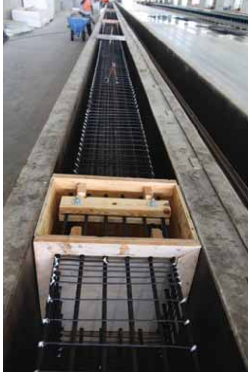
Figure H.26: CFCC strands, spirals, and wooden headers in position; ready to cast
