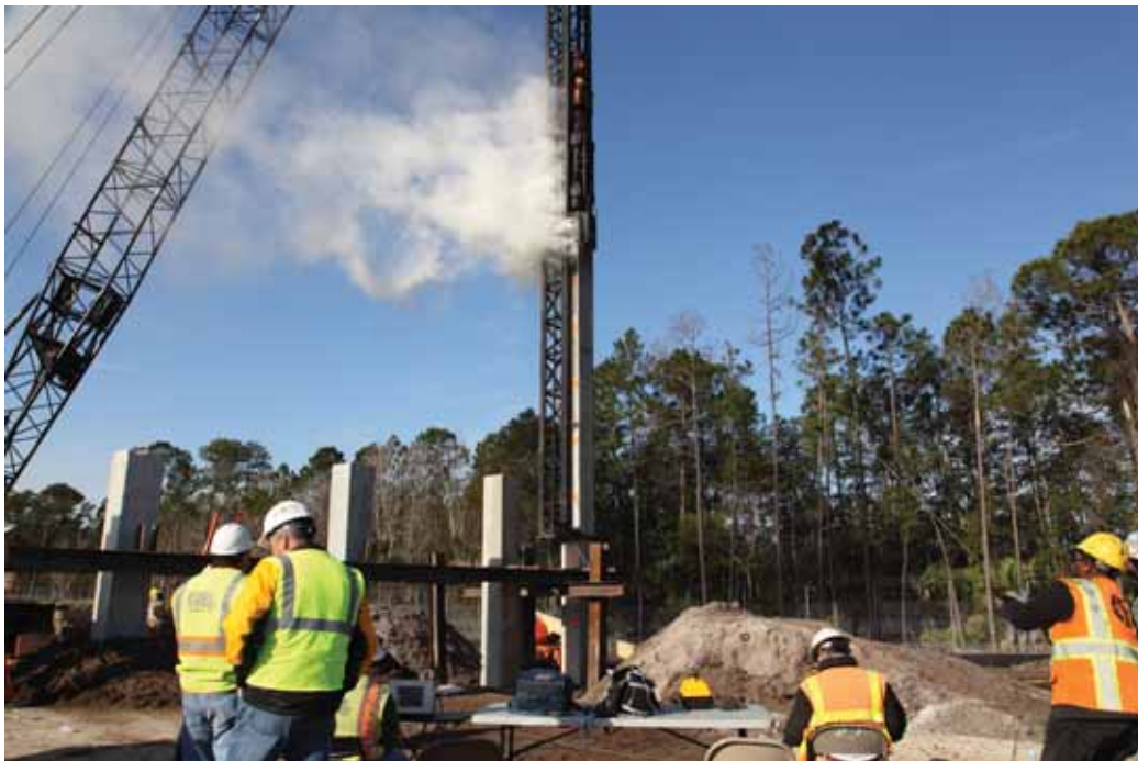
Figure H.36: Smoke during Pile 2 driving
