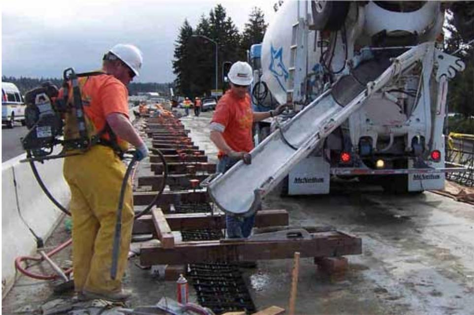
**Figure 1-1. Casting the closure region between phases.**
