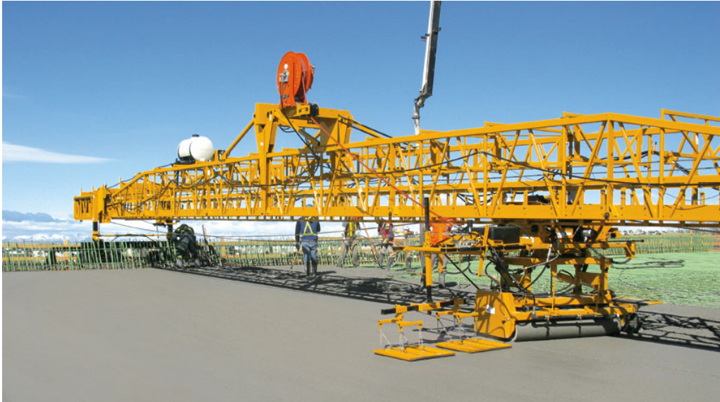
Figure 2.14 Typical bridge deck finishing machine in operation (Photo credit: Gomaco)
