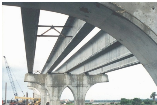
Figure 1.1 Prestressed concrete girders braced together for stability
