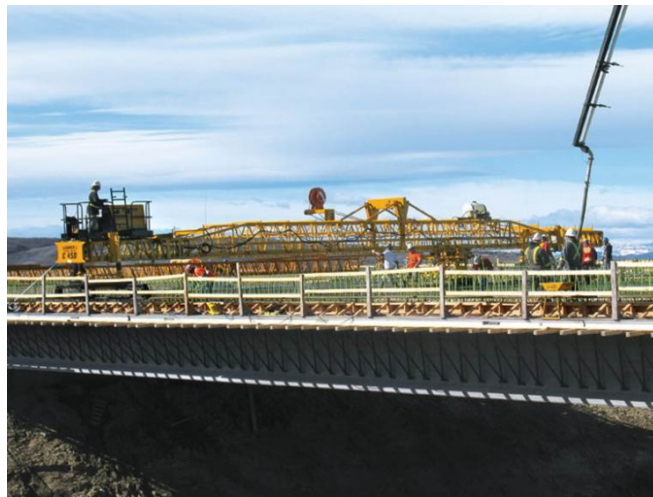
Figure 1.2 Bridge construction loads
