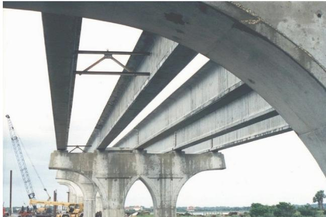
Figure 1.1 Prestressed concrete girders braced together for stability
