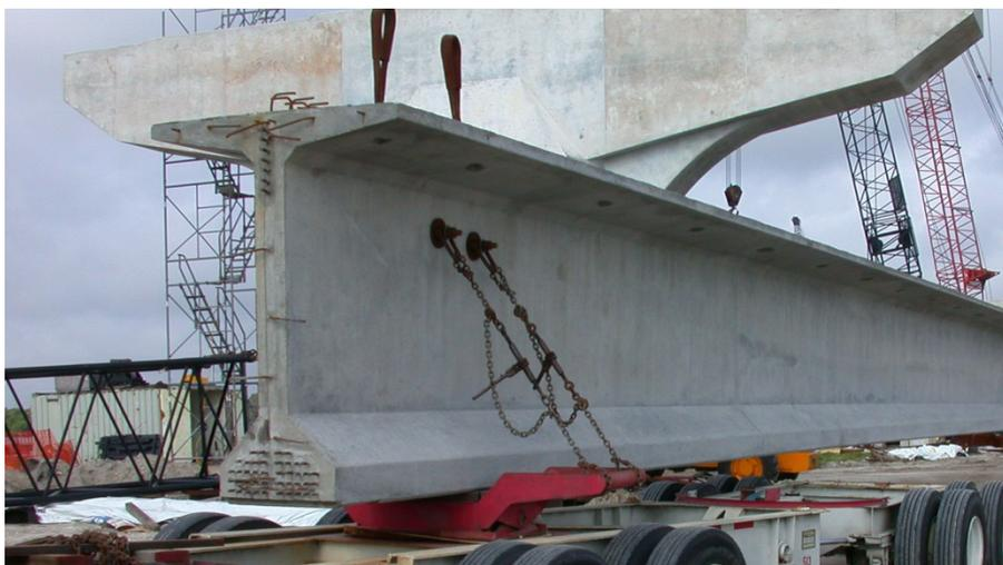
Figure 2.12 Chain braces on Florida Bulb-Tee during transportation
