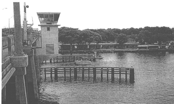
Figure 1.1. Fender Systems Currently Used by FDOT
