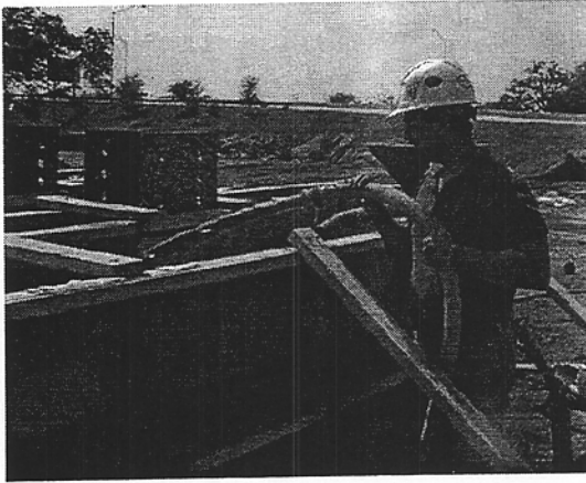
Figure 4.22 Filling Bentonite Bed.
