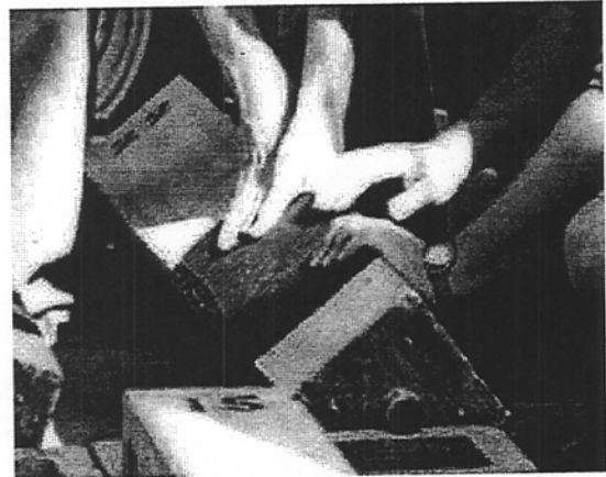
Figure 2.6 Placing Felt Paper.
