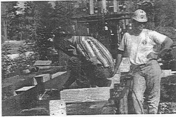
Welding the Steel Forms
