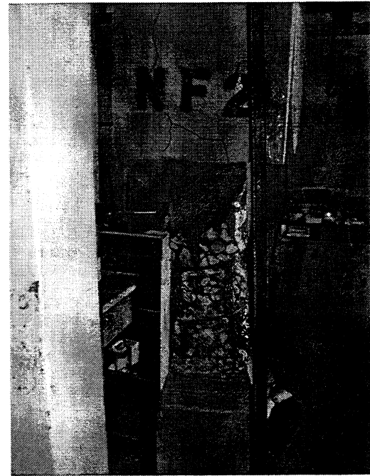
Note Buckling of Failed Strand
