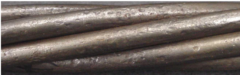
Figure 4 Condition of Strand- 35 days
