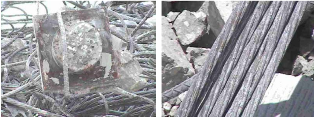
Figure 7.25 and 7.26 – Post-tensioning anchor and strands
