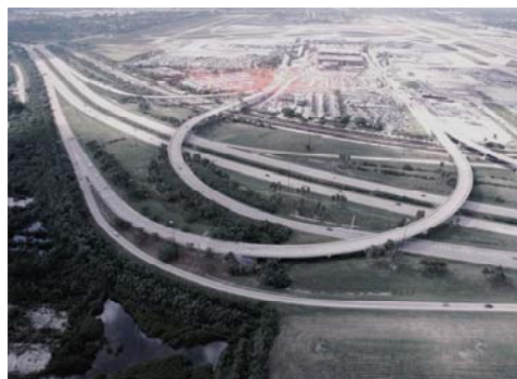
Figure 1.1 - Aerial photo of the Fort Lauderdale-Hollywood International Airport before Expansion. Ramp D Bridge is shown at the left above U.S. 1.
