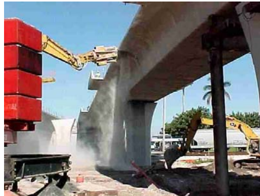
Figure 7.2 – Cutting the closure pour at mid span with the concrete crusher
