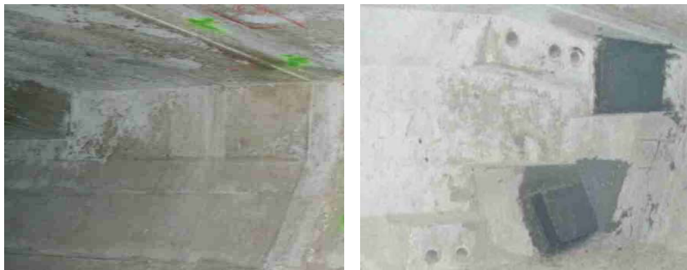
Figure 7.15 and Figure 7.16 – Segment joint and post-tensioning pourbacks
