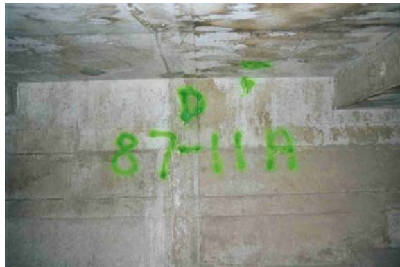
Figure 6.2 – Location at the inside of the Box for X-Ray inspection
