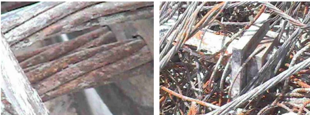
Figure 7.29 and 7.30 – Surface corrosion on remains after exposure to environment
