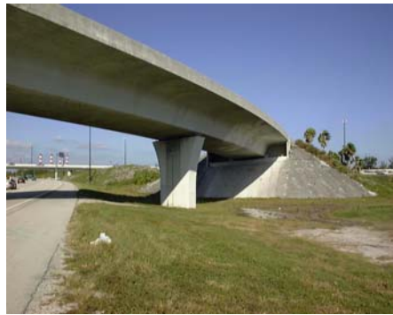
Figure 1.2 - View of Ramp D Bridge Span 6 over U.S. 1.
