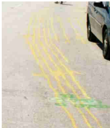
Figure 5.7 – Spray painted tendon paths
