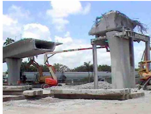
Figures 7.6 and 7.7 – Details of concrete crusher demolition method
