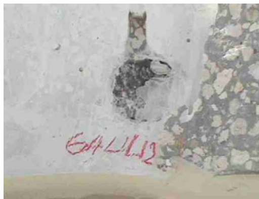
Figure 7.39 - Endoscopy inspection location not penetrating duct
