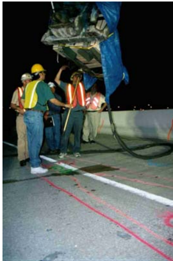
Figure 6.3 – Linear Accelerator suspended by the forklift
