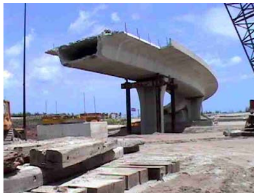
Figure 7.1 – View of a partially demolished cantilever with wings saw cut.
