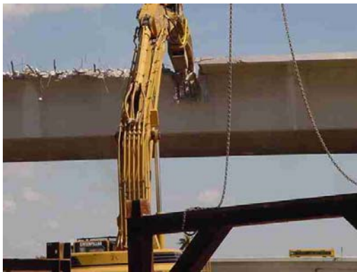
Figures 7.4 and 7.5 – Details of concrete crusher demolition method
