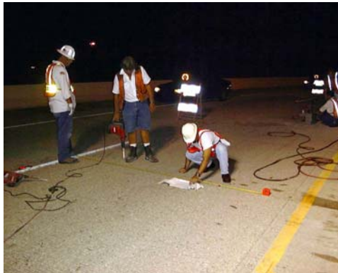
Figure 2.4 – Locating the tendons in the top deck
