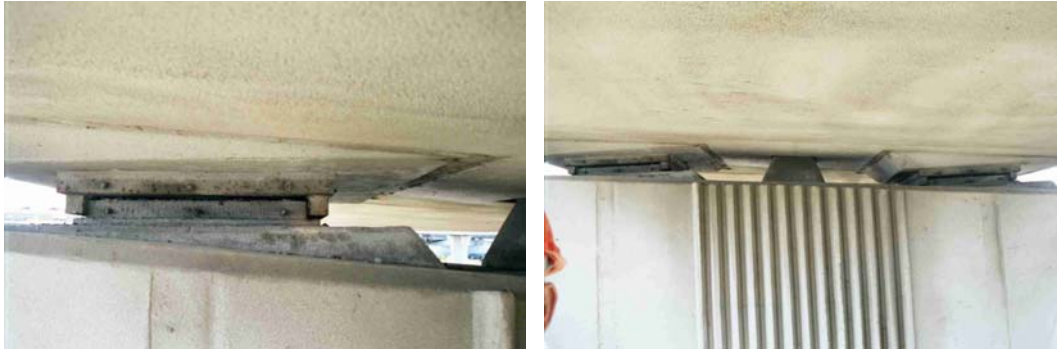
Figure 7.17 and Figure 7.18 – Pot bearings at Pier 6
