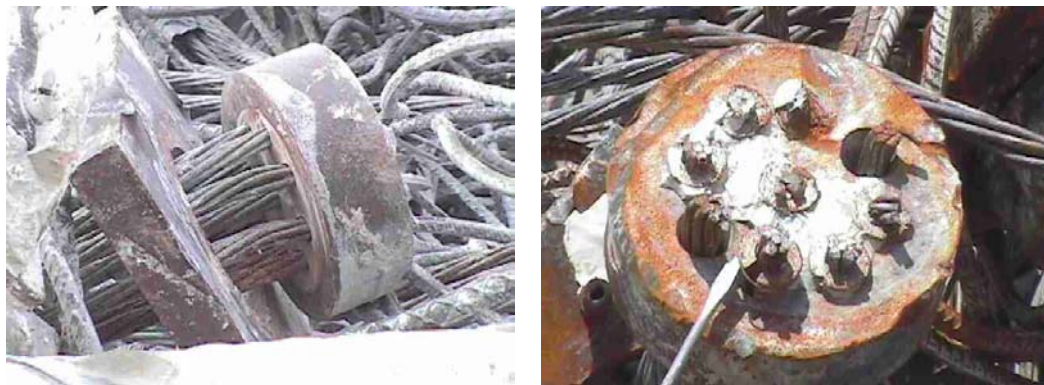
Figure 7.23 and 7.24 – Intact anchor systems in remains
