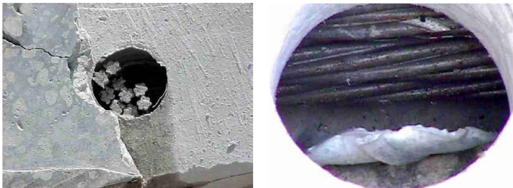
Figure 7.35 and 7.36 – UngROUTED tendon
