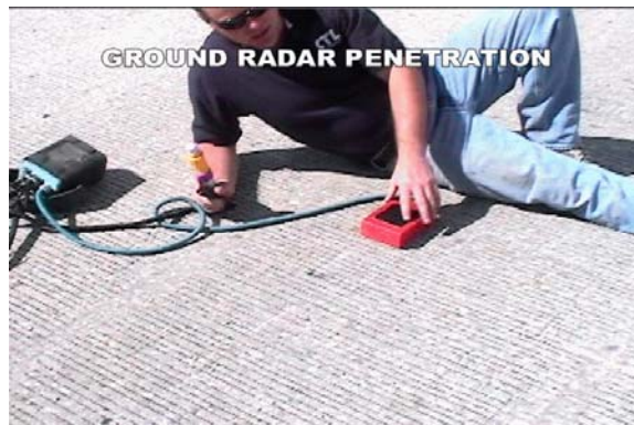
Figure 3.1 - Impulse Radar Testing
