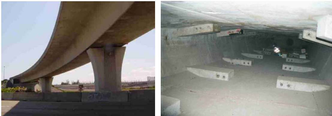
Figure 7.13 and 7.14 – Exterior and interior view of structure
