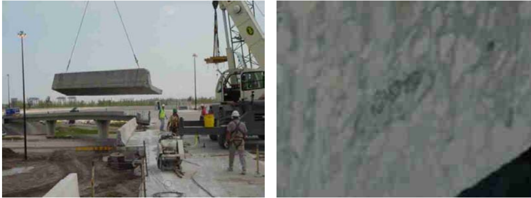
Figure 7.31 and 7.32 – Removal of portion of cantilever and transverse post-tensioning
