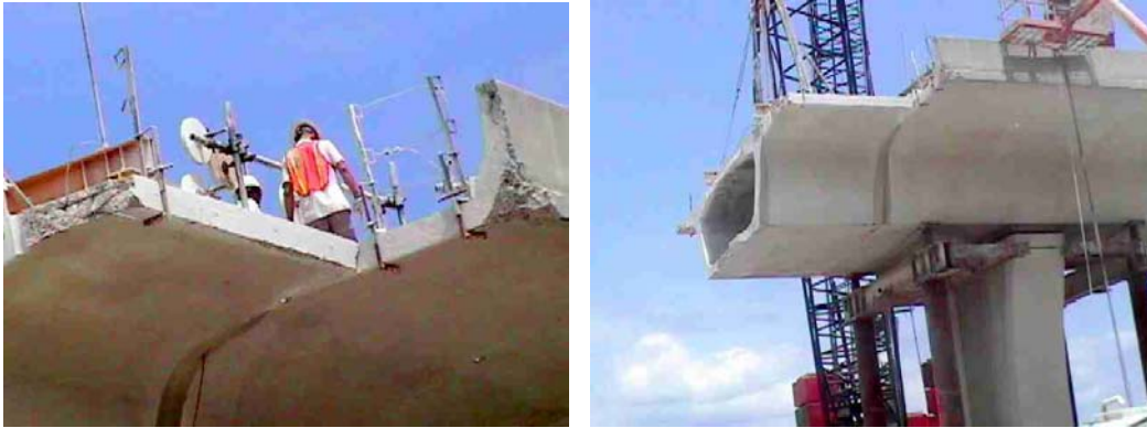
Figure 7.8 and 7.9 – Details of wire cutting demolition method
