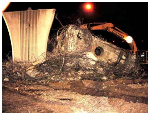
Figure 7.12 – Demolition of Span 7
