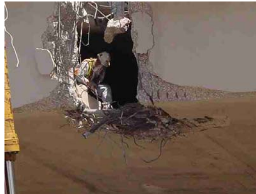
Figures 7.4 and 7.5 – Details of concrete crusher demolition method
