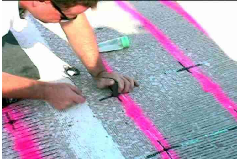
Figure 4.5 - Impact-Echo testing, impact application and receiver.
