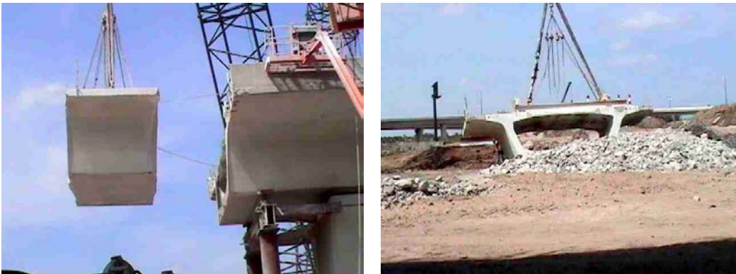
Figure 7.10 and 7.11 – Details of segment removal and storage
