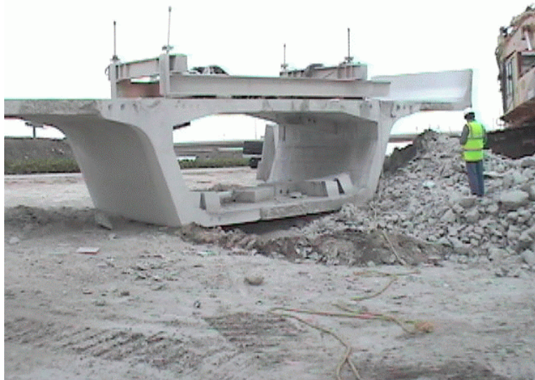
Figure 4.7 - Bridge segment after removal.
