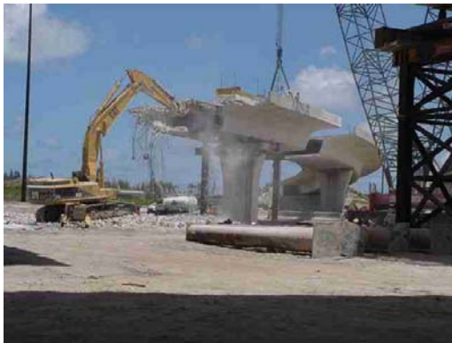
Figures 7.6 and 7.7 – Details of concrete crusher demolition method
