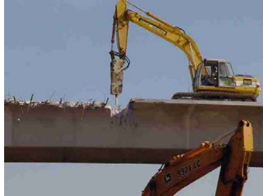
Figure 7.3 – Punching holes in top slab to facilitate concrete crusher machine operation
