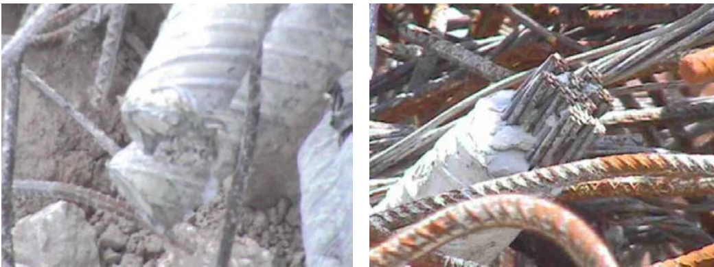
Figure 7.27 and 7.28 – Fully grouted duct with strands
