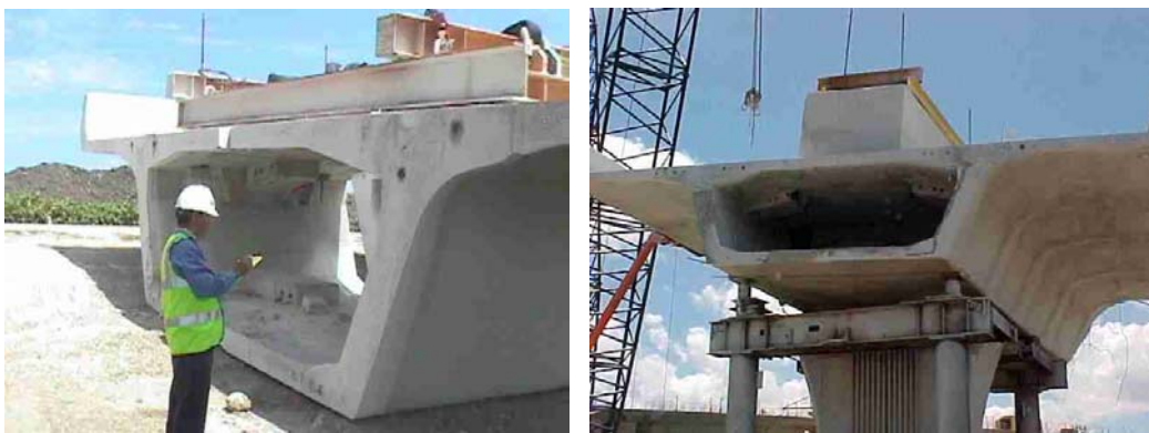
Figure 7.33 and 7.34 – Forensic inspection procedure showing voided ducts
