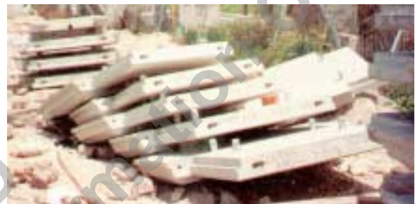
Figure 10, Improper Panel Storage
