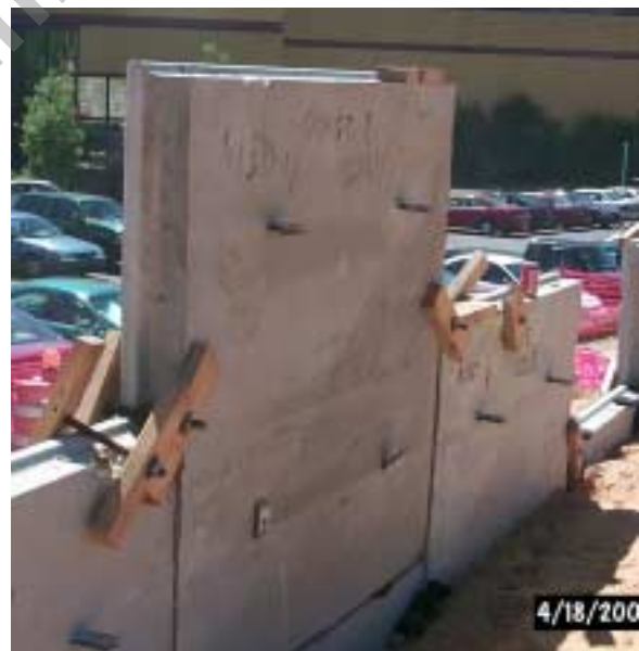
Figure 11, Damaged Tabs
