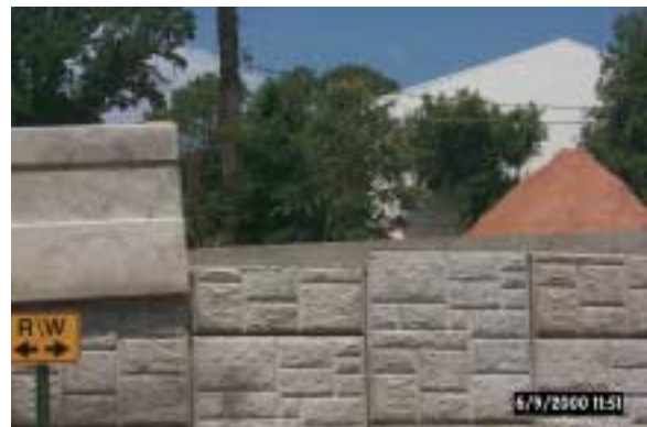
Figure 16, Leveling Course for Coping/Barrier
