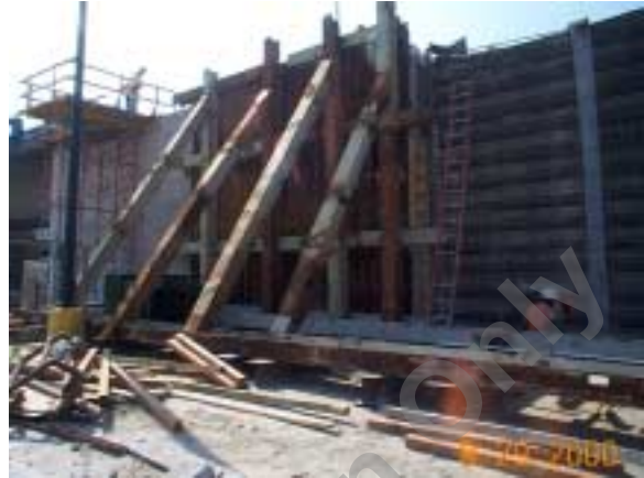
Figure 30, Temporary and Permanent Wall Facings
