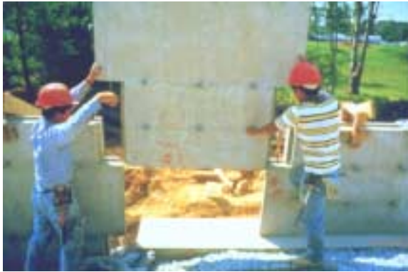
Figure 7, Placing Panels
