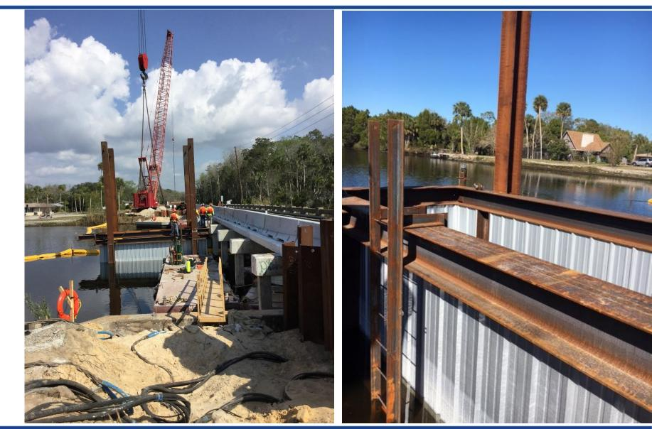
Driving 18" CFRP Concrete Pile
