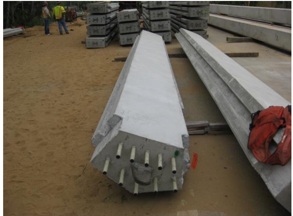
(Photographs - FDOT). Corner Sheet Piles stored on site
