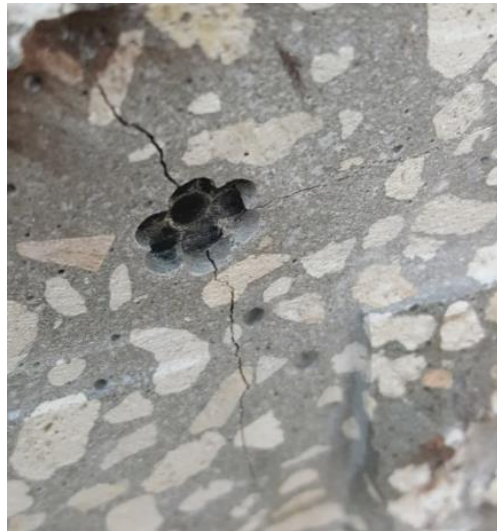
(Photographs - FDOT). Strand contraction and cracking at cut-offs.
