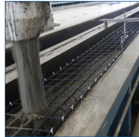
(photograph) FDOT. CFRP Pile Casting with SCC.
