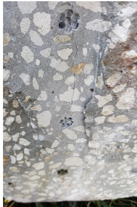
(Photographs - FDOT). Strand contraction and cracking at cut-offs.
