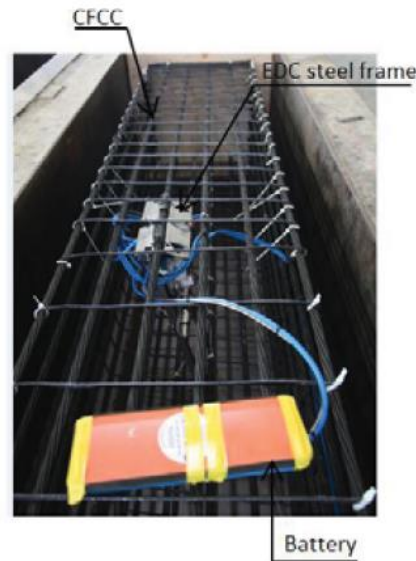
Figure 5.4: EDC installation
