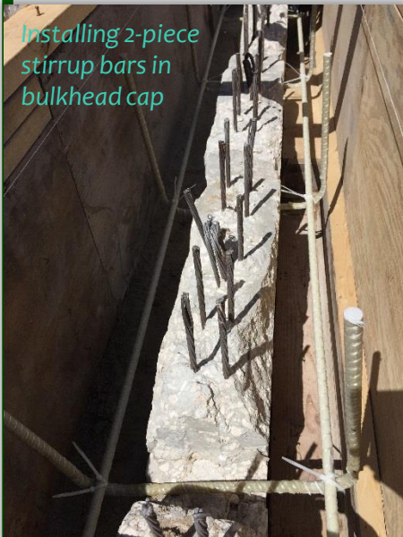
Installing 2-piece stirrup bars in bulkhead cap
