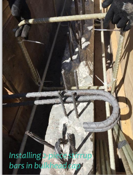
Forming bulkhead cap
