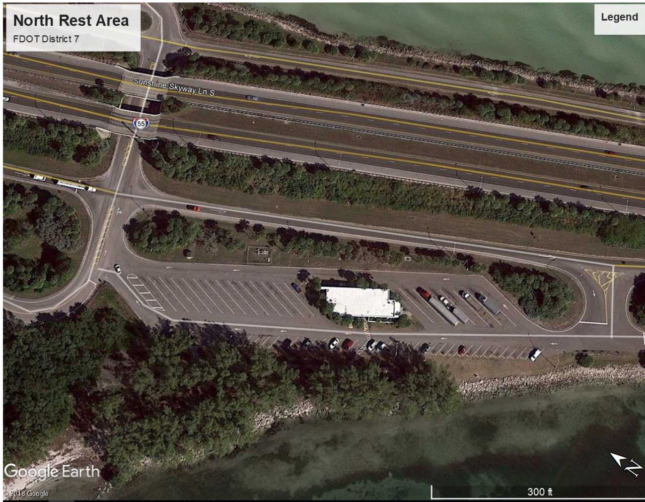
Existing North Rest Area
