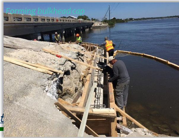
Installing 2-piece stirrup bars in bulkhead cap
