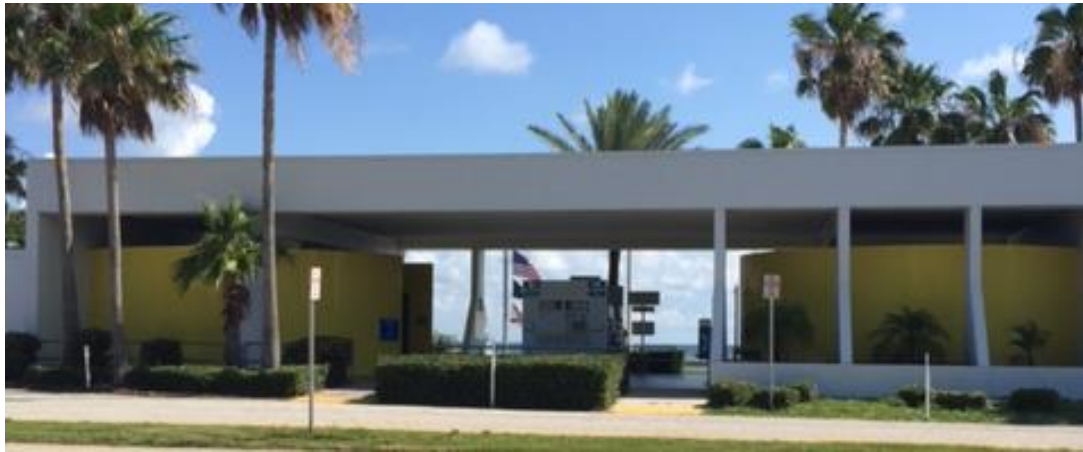
Existing Building (Manatee shown, Pinellas Similar)
