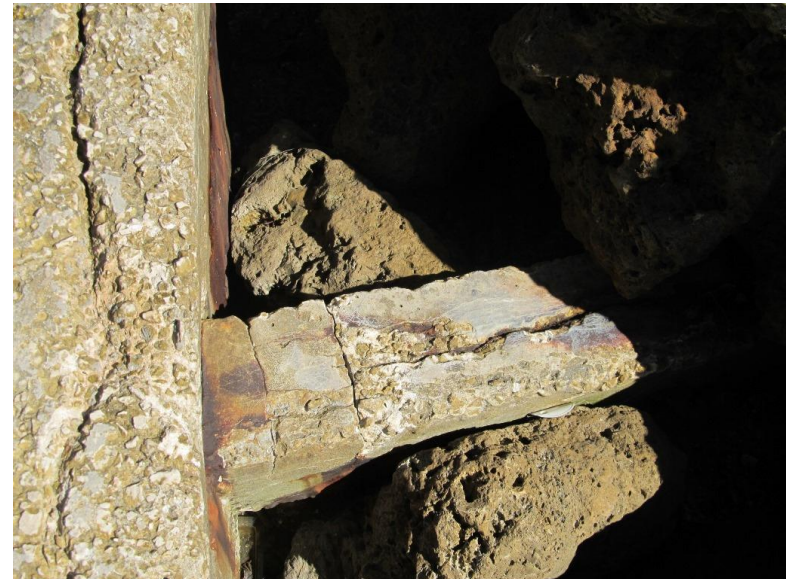
Northwest Area – Exposed Seawall Anchor
