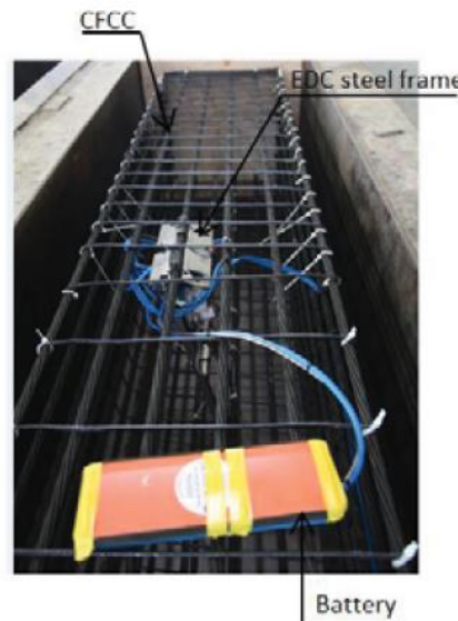
Figure 5.4: EDC installation
