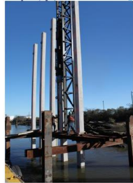
Figure 5.4 Driving of pile HSS #2
