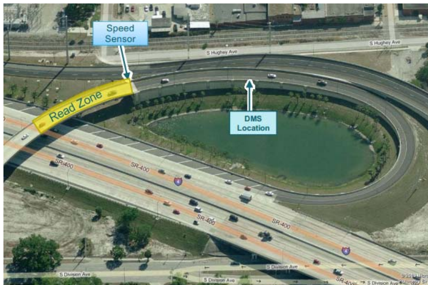
Overspeed Warning System on Loops
