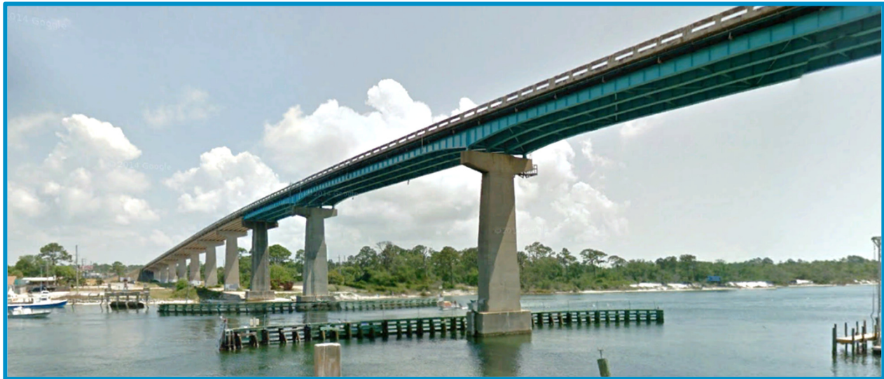
Source: "Perdido Key Bridge." 30°18'44.27" N and 87°25'36.41" W. Google Street View. Image capture May 2011.
