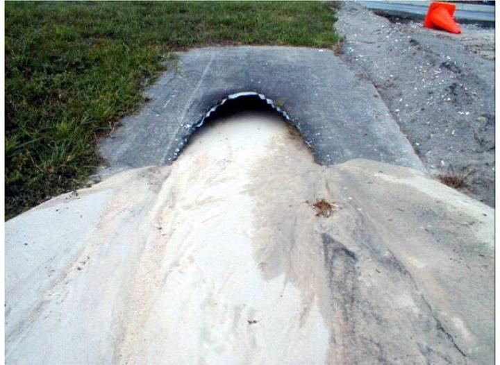
Uncontrolled erosion can result in blocked drainage systems.
