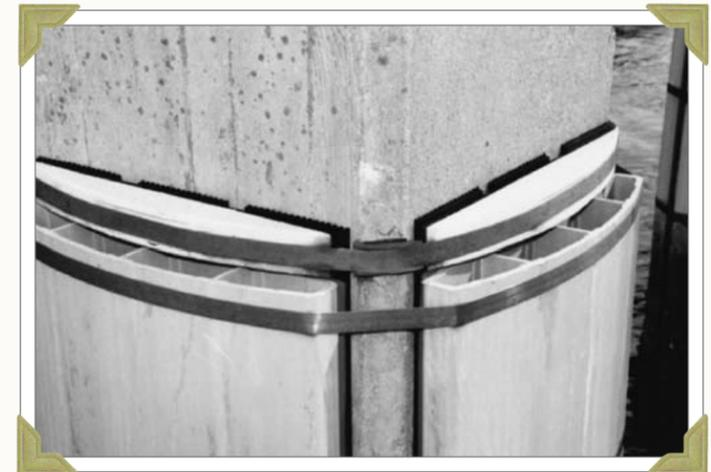
**Approx. 1987:** Conductive rubber was developed by FDOT and first used in 1987 on the piles of a bridge carrying US-90 in Jacksonville.
