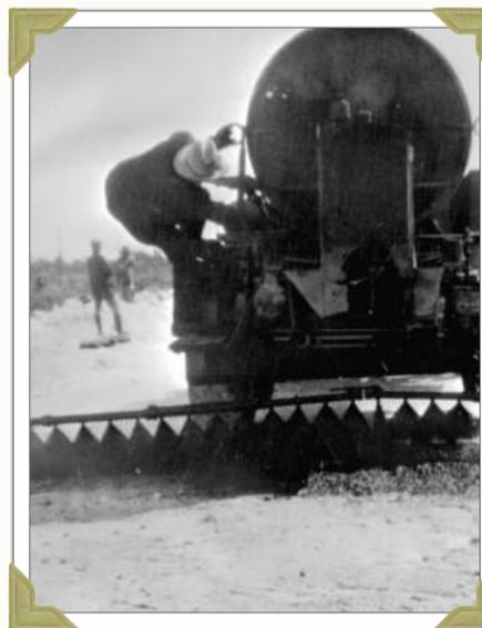
1917: Asphaltic oil is sprayed on a prepared roadbed to create a sand-asphalt road. Source: Florida Memory
