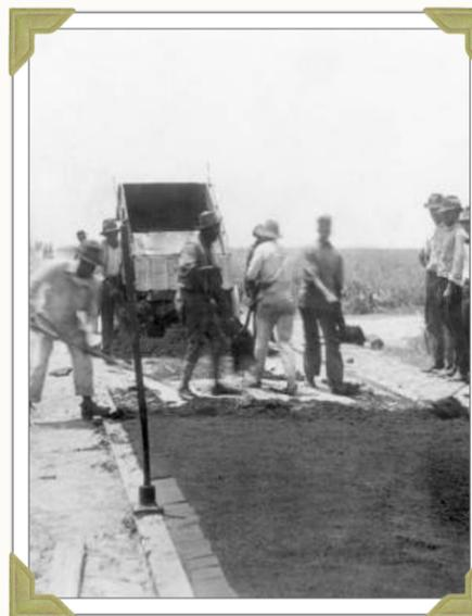
1917: A road crew lays base material in preparation for mixing and spraying for a new 9-ft road near Mulberry. Source: Florida Memory
