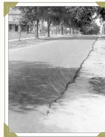
1917: A county-built sand-asphalt road near Mount Dora showing typical wear patterns and ragged shoulders. Source: Florida Memory
