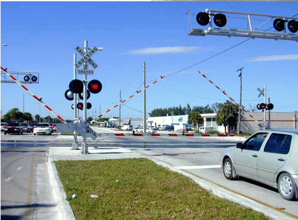
Exit gates descending.
