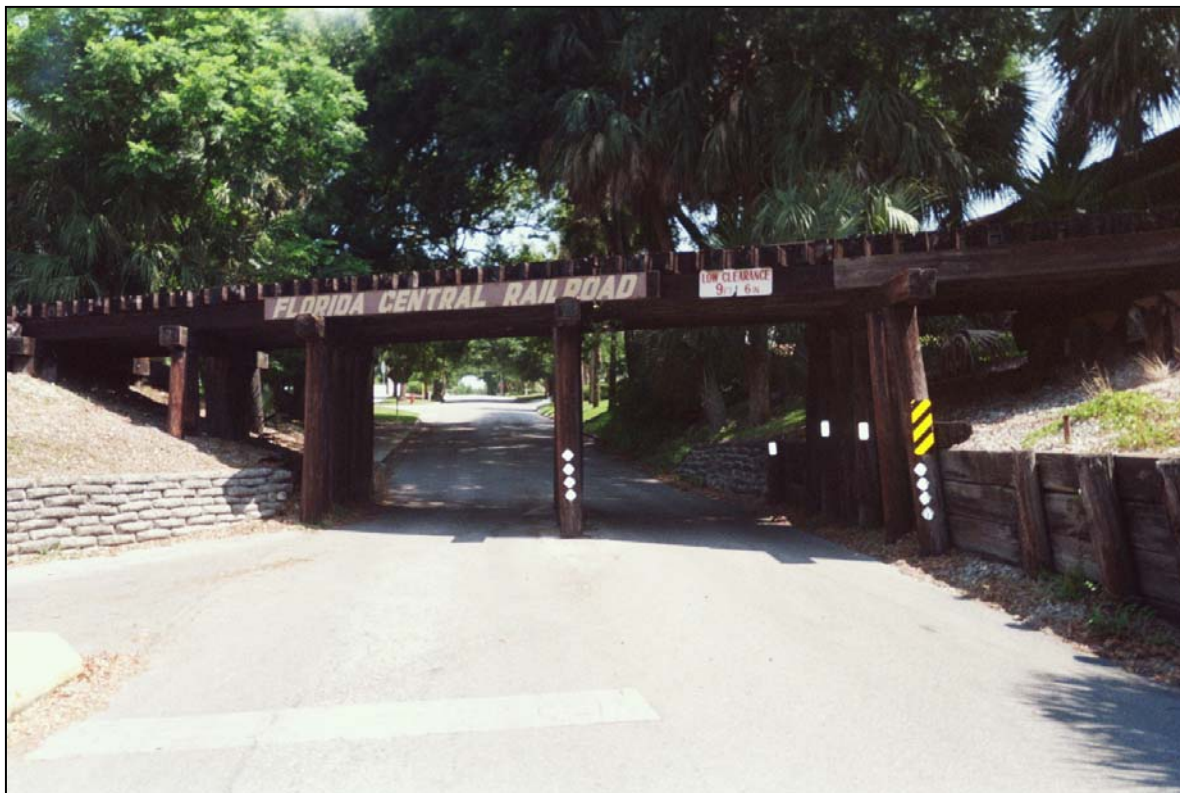
Figure 5.2 Railroad Bridge on the Florida Central
