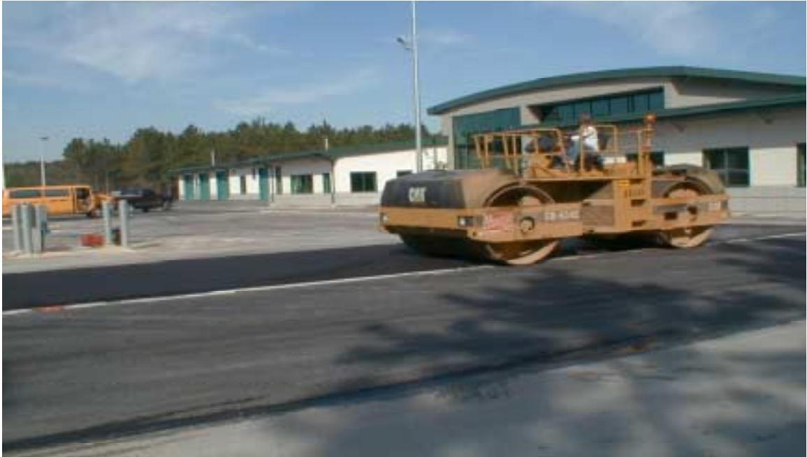
Figure 4.3 Photo of Steel-Wheel Roller Used for Compaction
