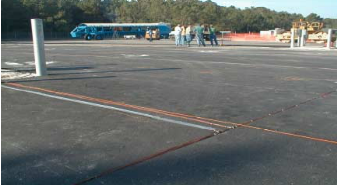
Figure 4.2 Photo of the Thermocouples Installed on the First Lift of HMA
