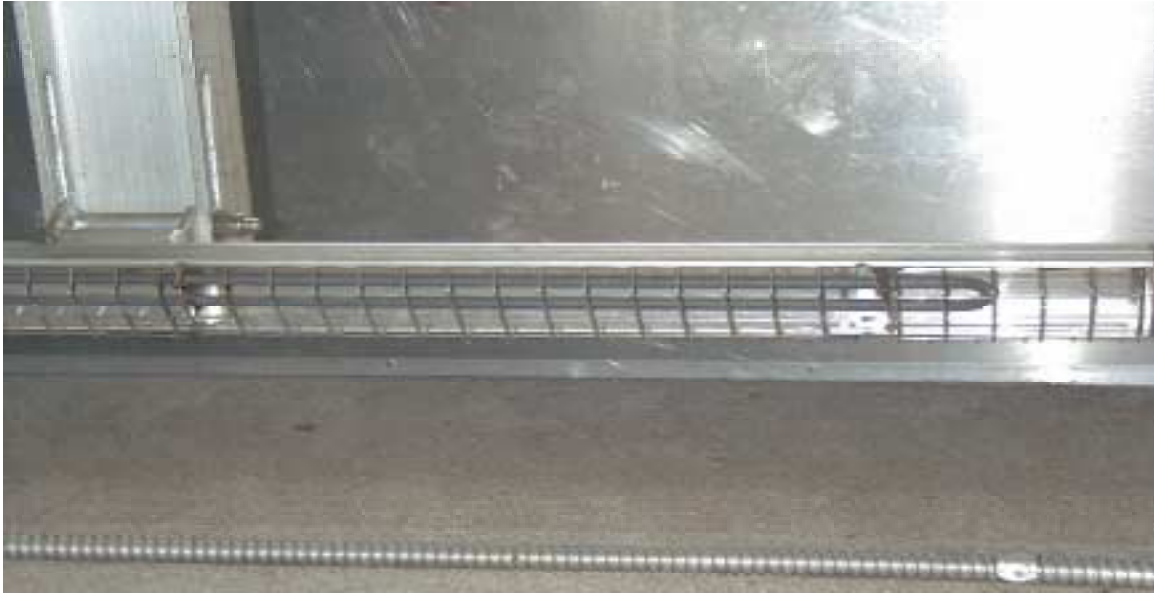
Figure 2.6 Photo of RAYMAX Hairpin Radiant Heater Unit
