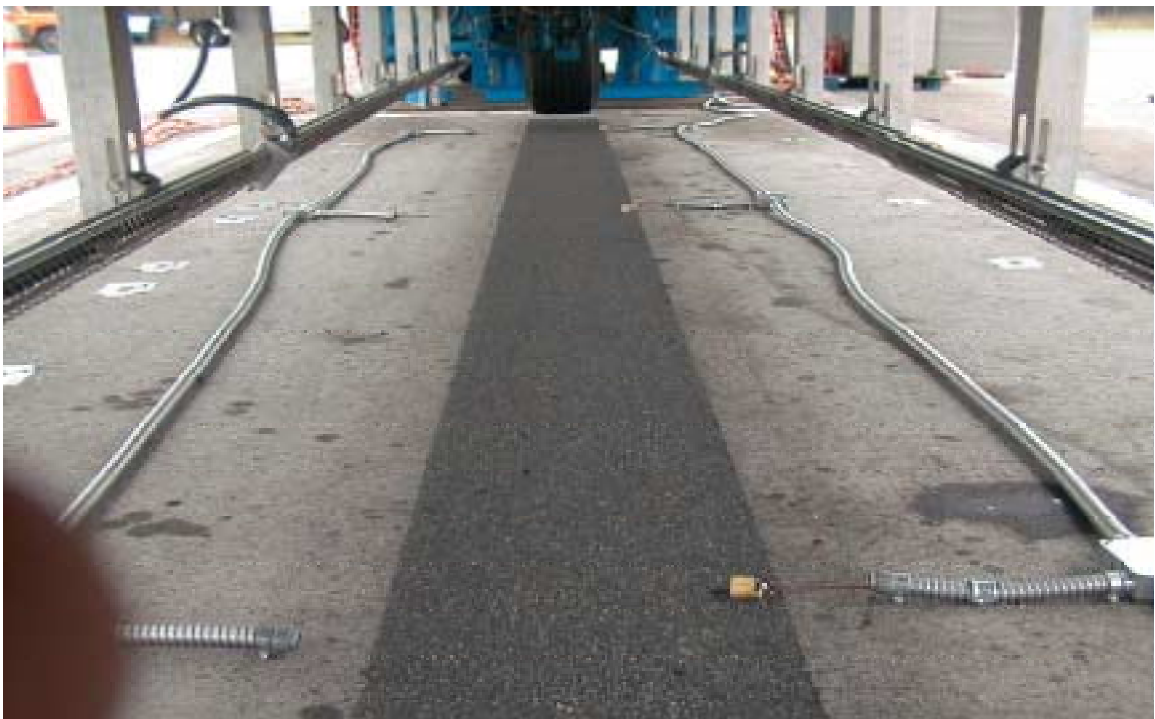
Figure 2.9 Photo of Pavement Inside of Insulating Area
