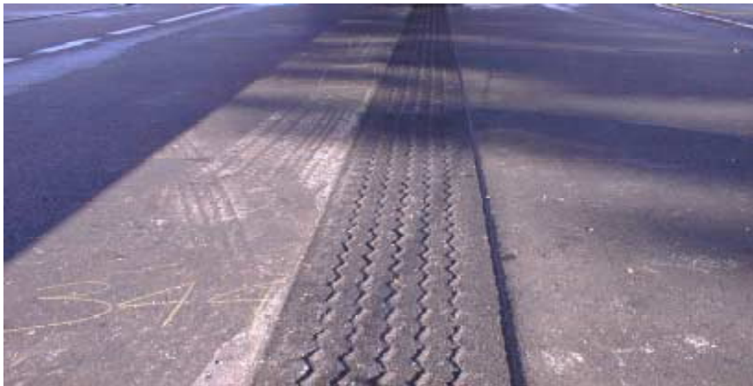
Figure 5.3 Photo of Section 7C
