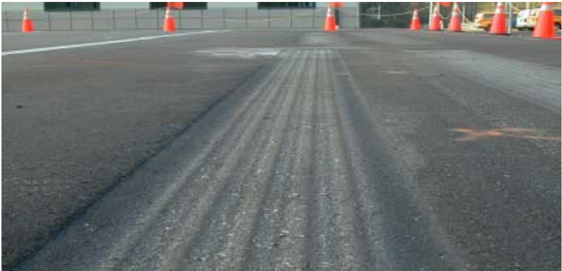
Figure 5.4 Photo of Section 7B-W
