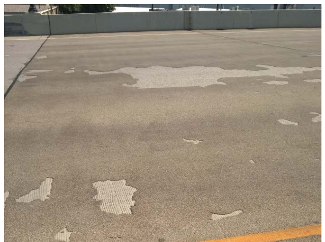
FIGURE 15 – Delamination.
