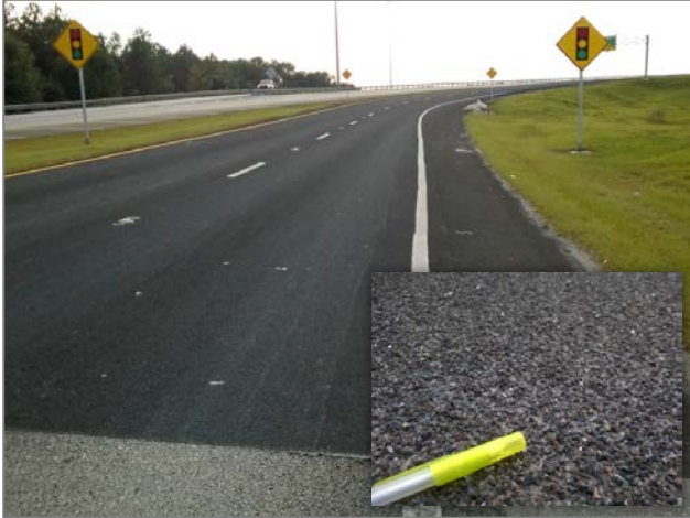
FIGURE 1 – High friction surface treatment.
