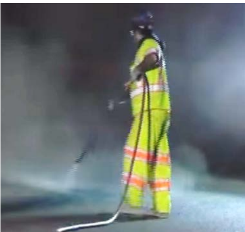
FIGURE 7 – Proper air wash technique.
