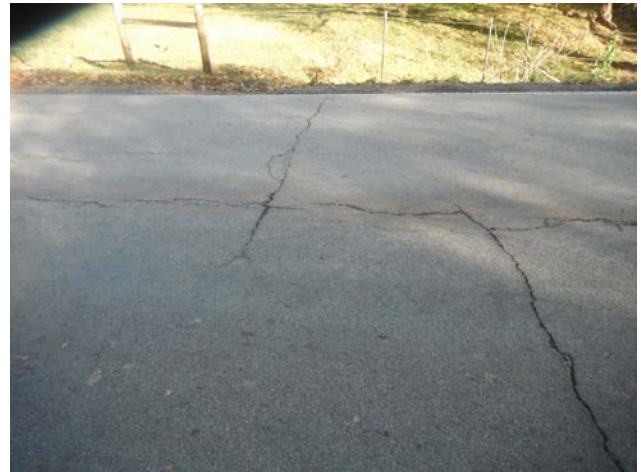
FIGURE 22 – Reflective cracking.
