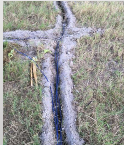
Step 3: Install sensor using CPT/SPT trucks
