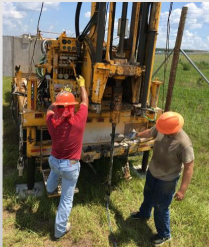
Step 2: Install sensor using CPT/SPT trucks
