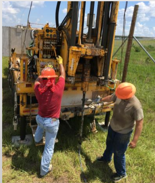
Step 2: Install sensor using CPT/SPT trucks
