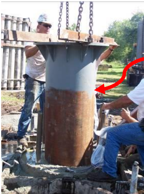
Pipe and flange connector (for combined torsion and lateral loading)
