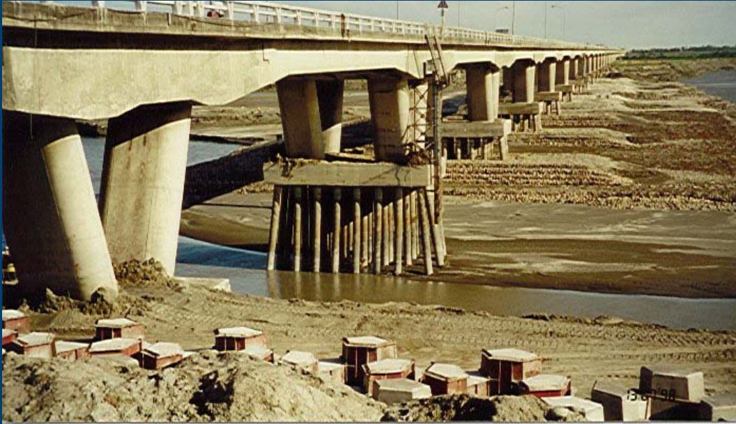
Bridge Scour Photograph
