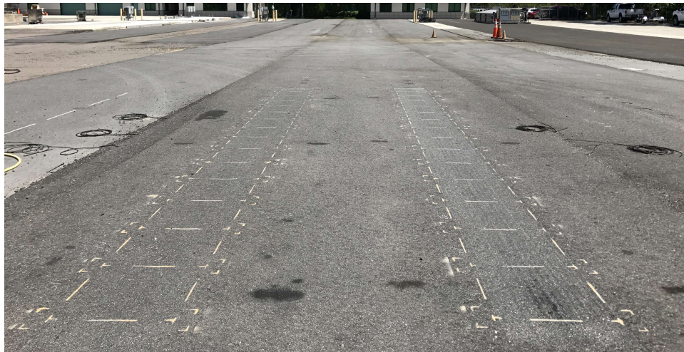
Figure 5. HVS Loading Area with Texture Measurement Segments
