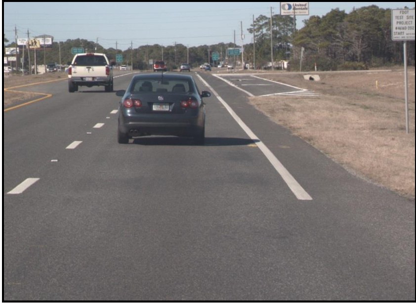
FIGURE 1. SR-30A at milepost 4.577
