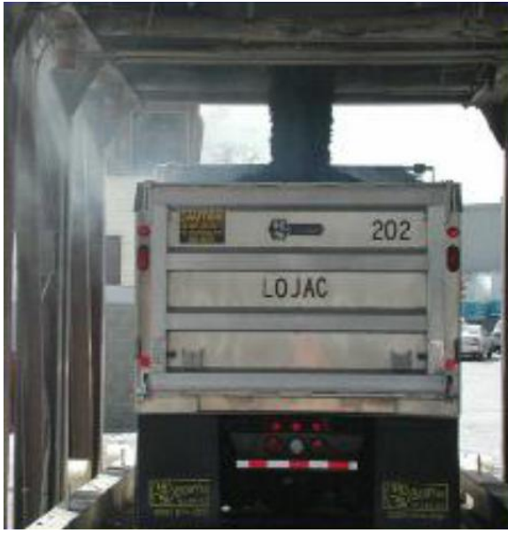
(a) Hot-Mix Asphalt (HMA) at 320 °F
