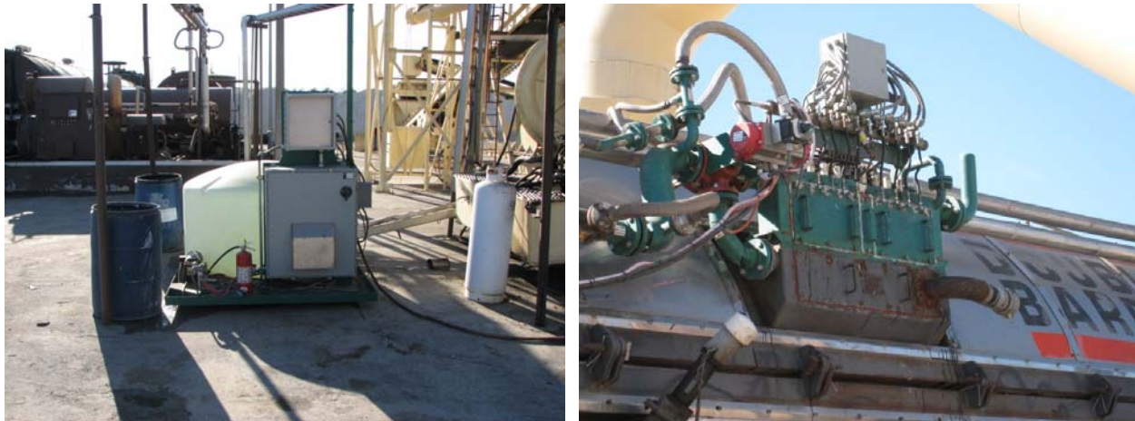
Figure 6 - Astec Double Barrel Green Warm Mix Process
