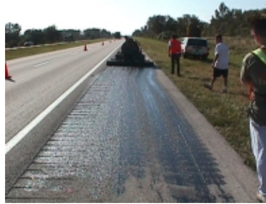
Figure 4 - Non-uniform Spray Pattern
