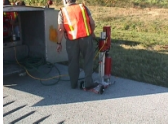
Figure 2 - Coring Pavement Prior to Treatment
