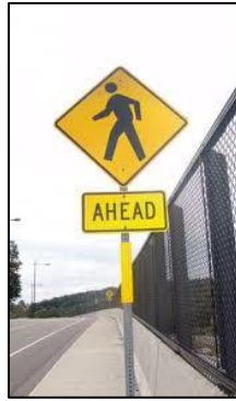
Figure 12: Example of a Reflective Sign Post Treatment
