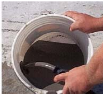
Figure 13, Discharging good grout from vent pipe
