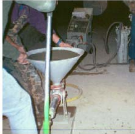
Figure 17. Vacuum grouting for Mid Bay Bridge repair
