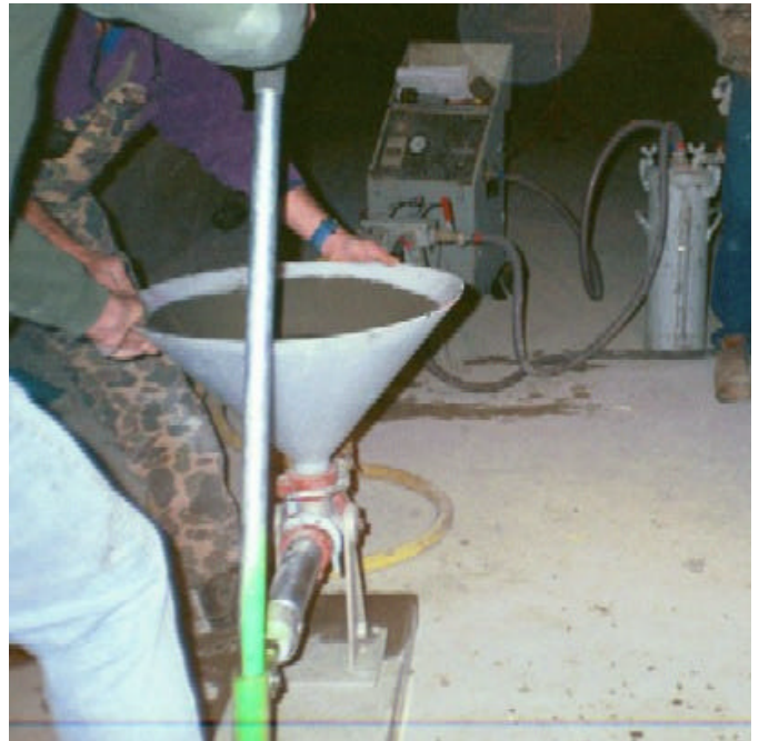
Figure 17, Vacuum grouting for Mid Bay Bridge repair
