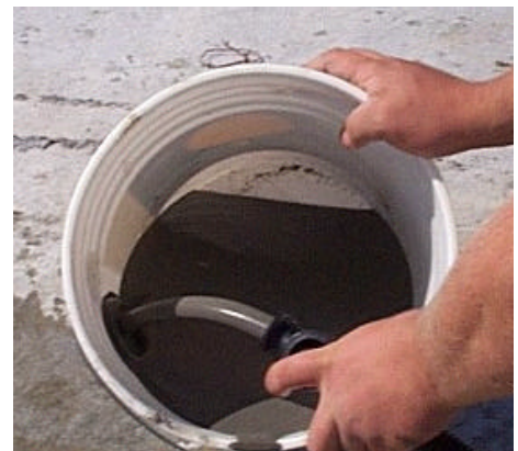
Figure 13, Discharging good grout from vent pipe
