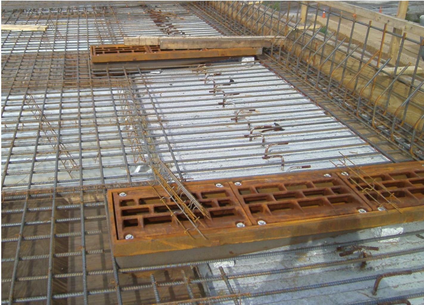
Embedded Drainage Structures Prior to Concrete Placement
