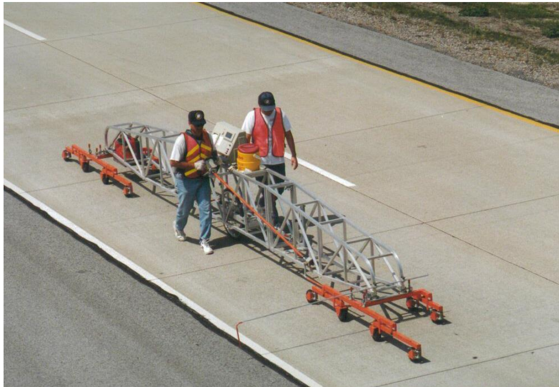
Profilograph Being Used on Concrete Pavement
