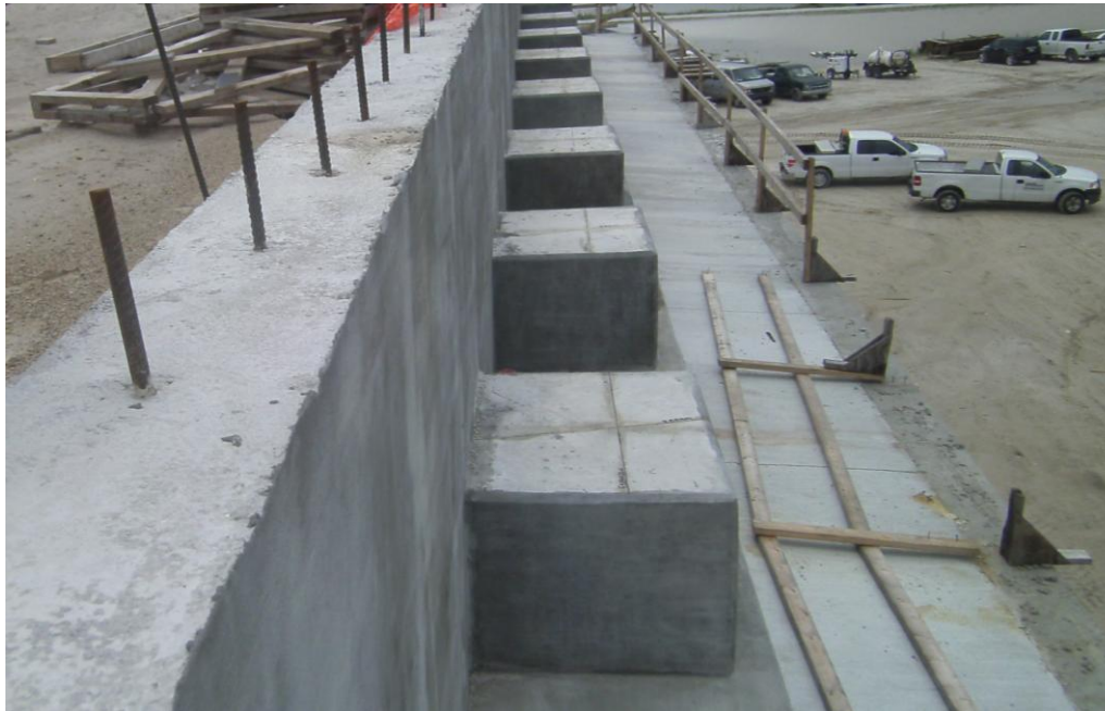
Beam Pedestals – Note the marks showing bearing and girder alignment
