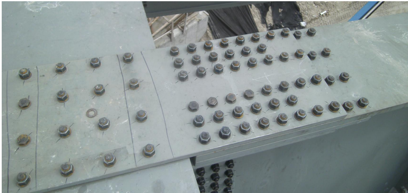
Splice Plate Connection – Note the markings where the “Turn of Nut” rotation was recorded
