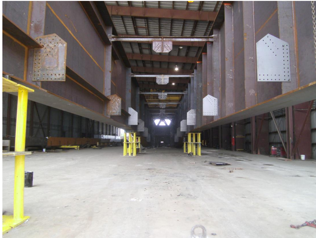
Steel Plate Girders at a Fabrication Facility
