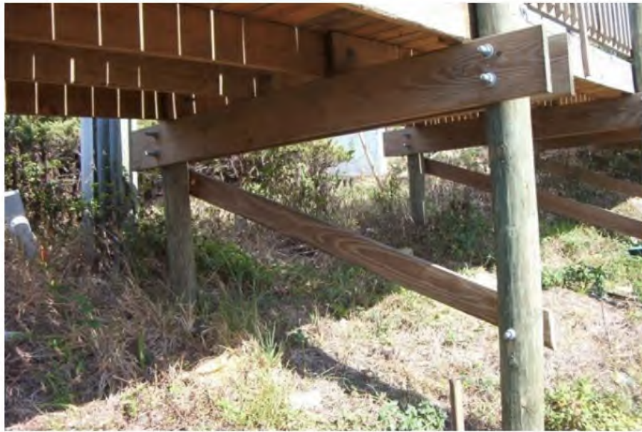
Support piling / post with bracing.
