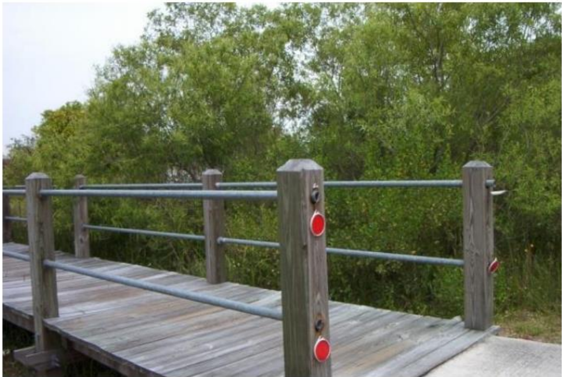
Pipe handrail
