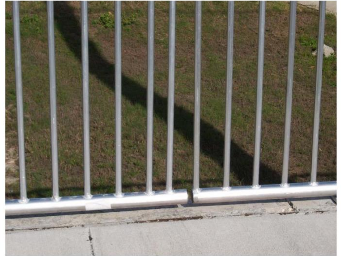
Picket railing missing steel sleeve at expansion joint. This does not meet MRP standards.
