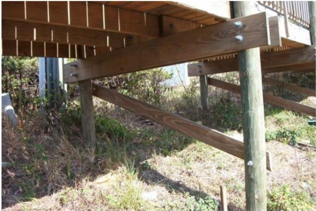
Support piling / post with bracing.
