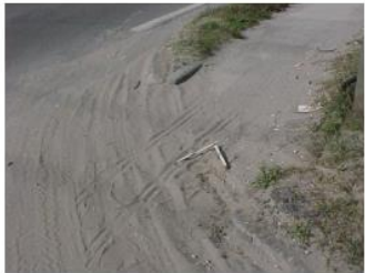
These pictures show example of sand buildup on sidewalk. Sweeping should be rated around the area.
