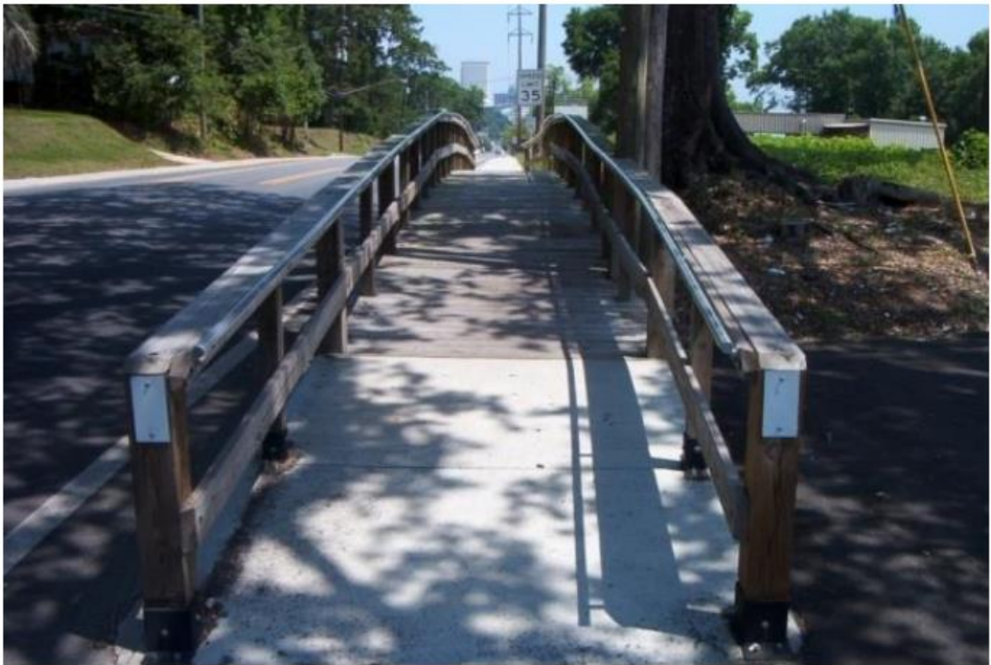
Wood with pipe handrail
