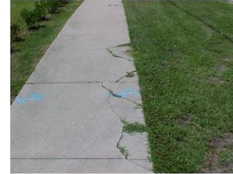
Sidewalk cracking. Measure each horizontal crack greater than \frac{1}{2} inch wide. For MRP purposes, each linear foot of horizontal crack greater than \frac{1}{2} inch equals 1 sq. ft. of crack area. Vertical misalignments greater than \frac{1}{4} inch equals 1 sq. ft. of crack area.
