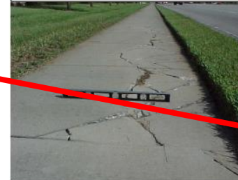
Sidewalk cracking. Measure each horizontal crack greater than \frac{1}{2} inch
