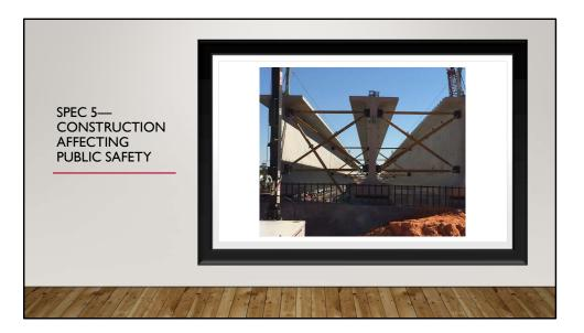
Here we have a good field shot of the beam end and intermediate temporary bracing scheme for three FIB girders.
