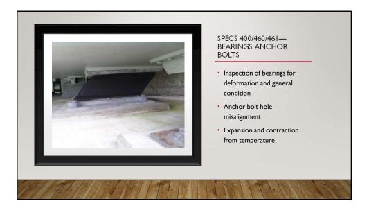
Other things we look for are bearing deformation and general condition, anchor bolt misalignment.
