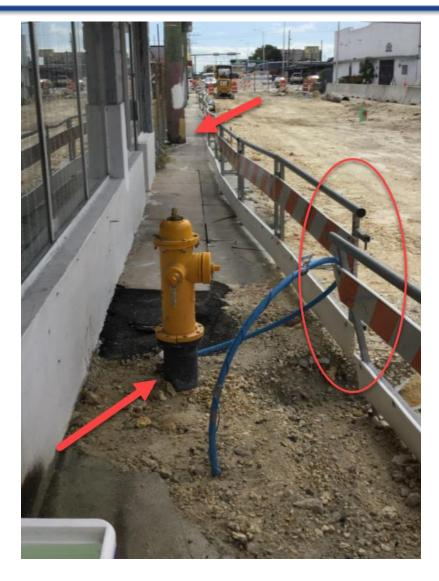
Pedestrian walkway was not properly detoured and Ped LCDs were not properly maintained. Index 102-660 and ADA Guidelines require <u>all temporary</u> walkway surfaces be accessible with firm, stable, slip resistant and kept free of obstructions. Spec 102-9.5.2 also requires joints between Ped LCDs must a maximum offset of 1/2 inch in any one plane.
