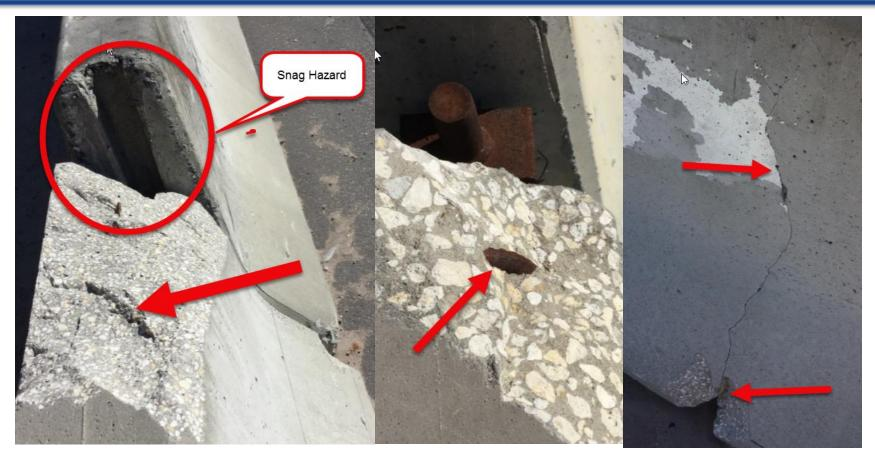
**Type K barrier contained significant cracks throughout the cross section and large spalls with exposed rebar.** Spec 102-9.1 requires all temporary concrete barrier to meet acceptable standards as outlined in the Department's Temporary Concrete Barrier Evaluation Guide.
