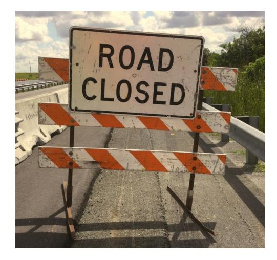
**Type III barricades** were not properly maintained. Specification 102-9.1 requires all temporary traffic control devices to meet Acceptable standards as outlined in the ATSSA's **Quality Guidelines for** Temporary Traffic Control **Devices and Features**.
