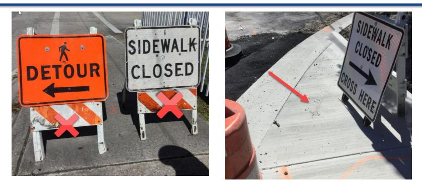
Type II barricades with signs attached used to close sidewalks and curb ramps did not have detectable warnings. Index 102-660 requires pedestrian <u>LCDs be placed across the</u> <u>full width of closed sidewalks</u> and requires curb ramps to have <u>detectable warnings</u>.
