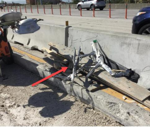
**Construction debris, stockpiled material and other objects within deflection space of Type K barrier.** Index 102-100, Sheet 1 requires the <u>deflection space to be clear of any grass, construction debris, stockpiled</u> <u>materials, equipment and objects</u>.
