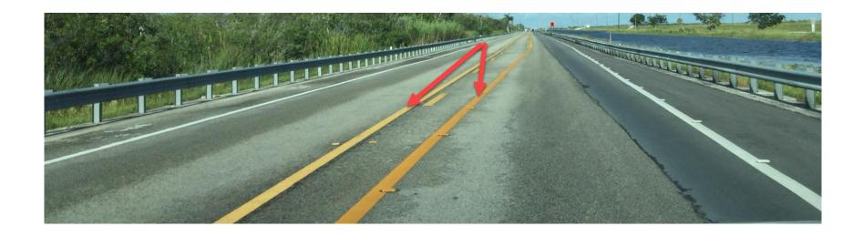
One area of the project had conflicting pavement markings. Index 102-600, Sheet 8 requires the removal of existing pavement markings that conflict with temporary work zone delineation when work exceeds one daylight period.
