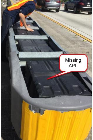
**Crash cushions** missing APL number. Spec 102-9.1 requires the APL number to <u>be</u> permanently marked on all TTC devices at a readily visible location.
