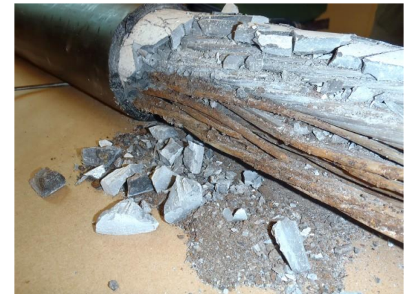
Post-Tensioning Grout (SS 938)
