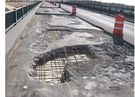
Materials for Concrete Repair (SS 930)
